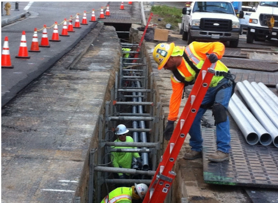
Conduit Installation for DWP Power at 2 nd St. and Hope
