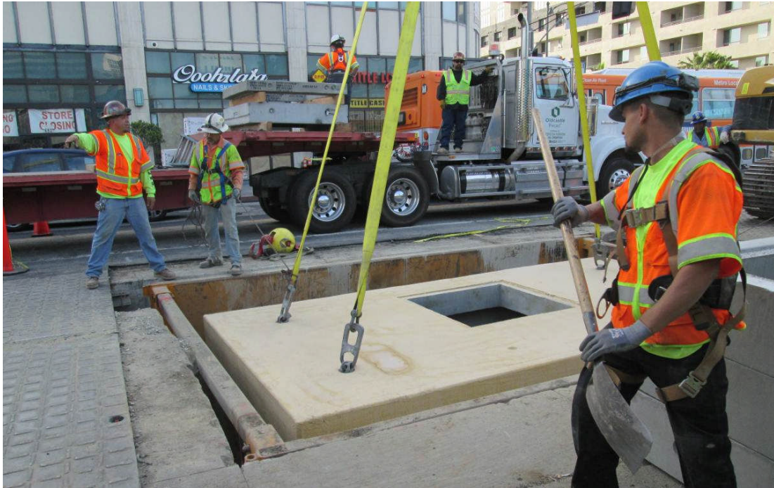
LADWP Power Vault 677 Upper Section Being Installed
