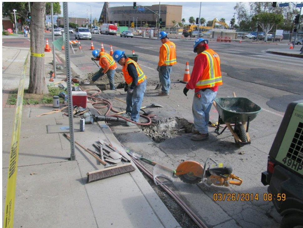
Potholing on Crenshaw Boulevard near Rodeo Street.
