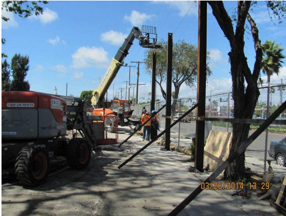
WSSC installation of I-beams for noise wall installation at Expo Station site.
