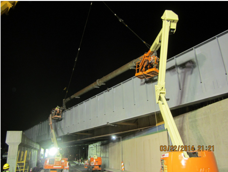
Segment 4: Foothill Bridge - Steel Girder Erection
