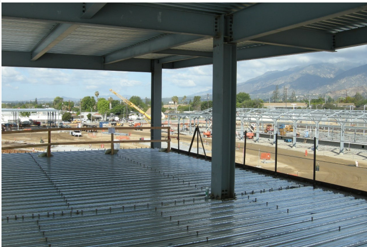
Operations Campus: 3rd floor Yard Control Room decking complete
