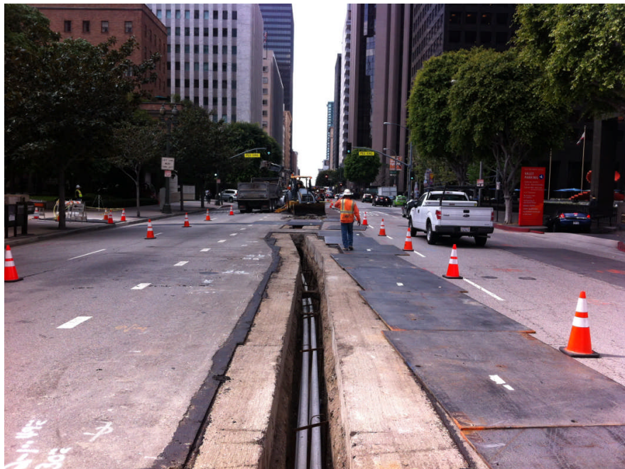
5 th Street and Flower – AT&T CA Pipe installation
