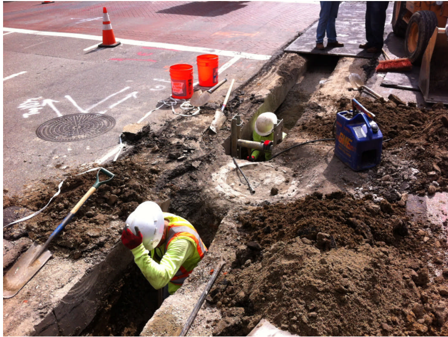
5 th Street and Flower – use of shoring for TWC facilities
