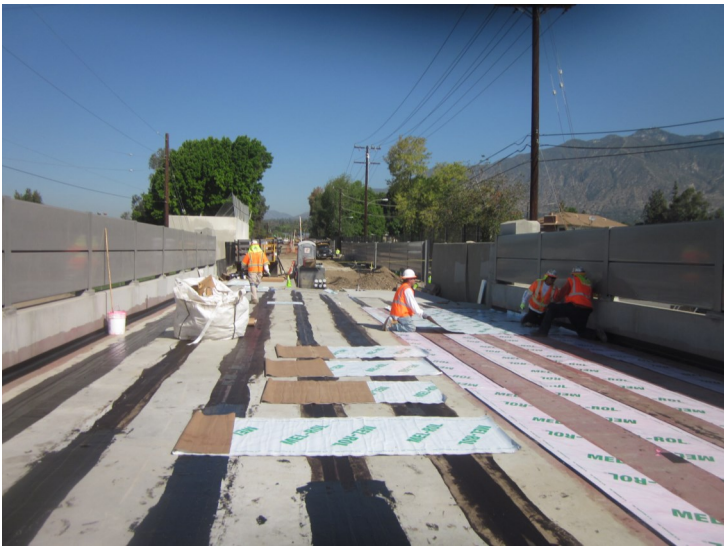
Segment 2: Colorado Bridge Waterproofing
