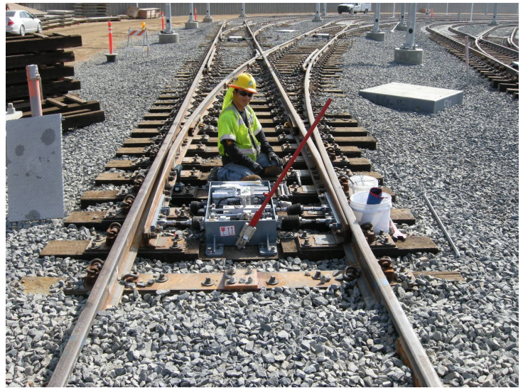
Operations Campus: Track Switch Installation
