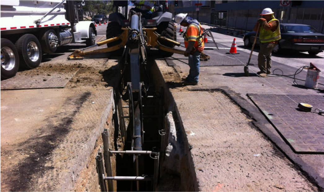
Trenching continuation for the DWP Power at Hope Street
