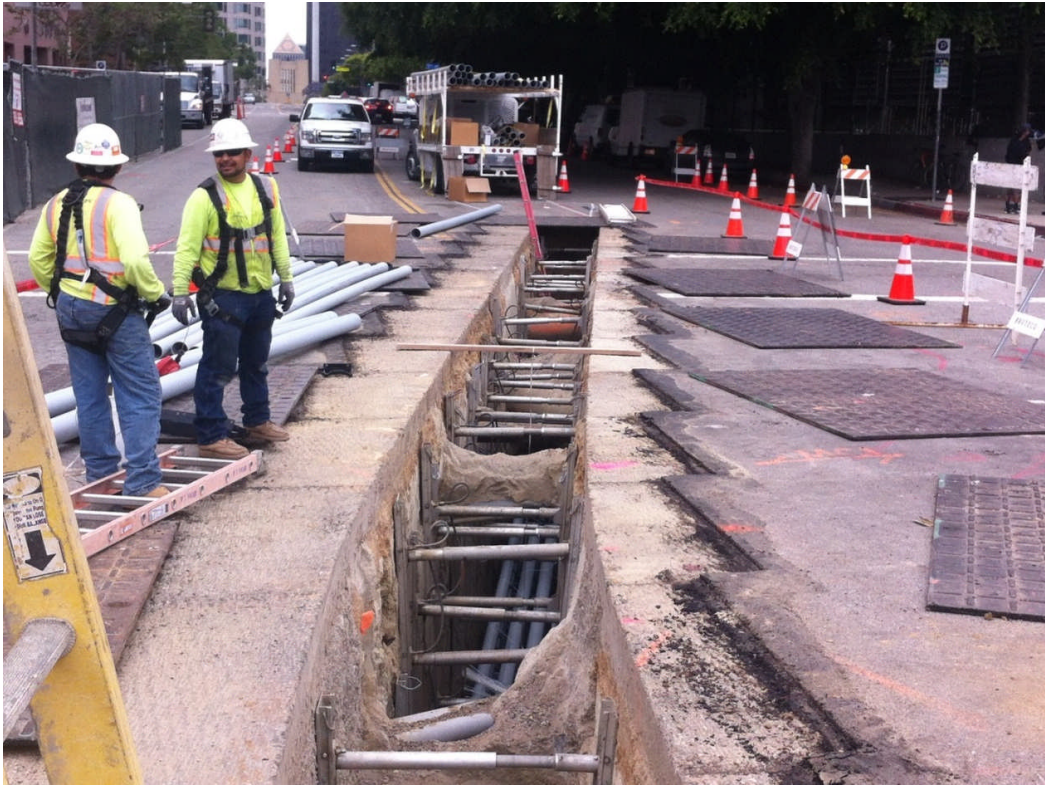
Conduit Installation for DWP Power at Hope Street
