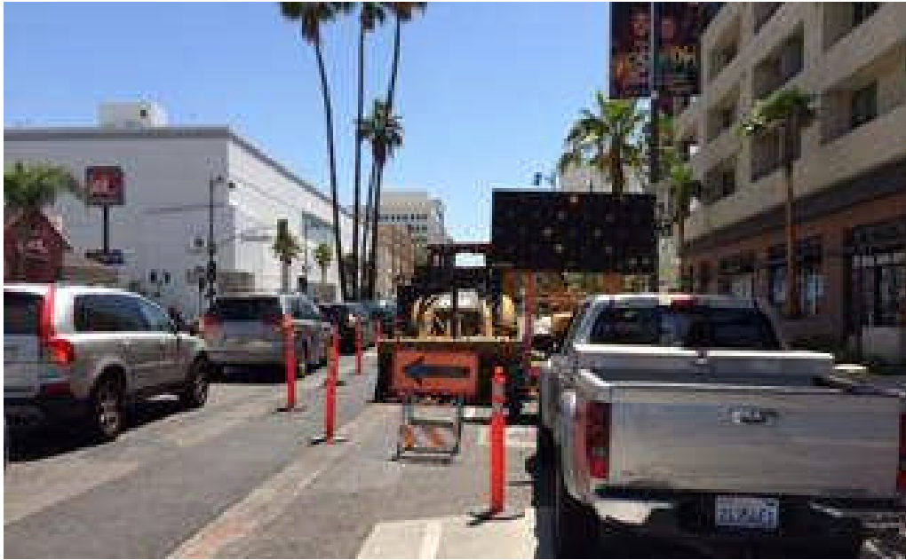
Traffic control equipment for AUR lane closure near Wilshire/La Brea intersection.
