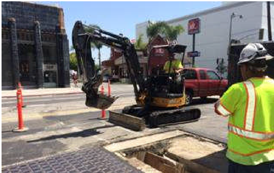
C1048 contractor making use of compact excavator to minimize traffic impacts.
