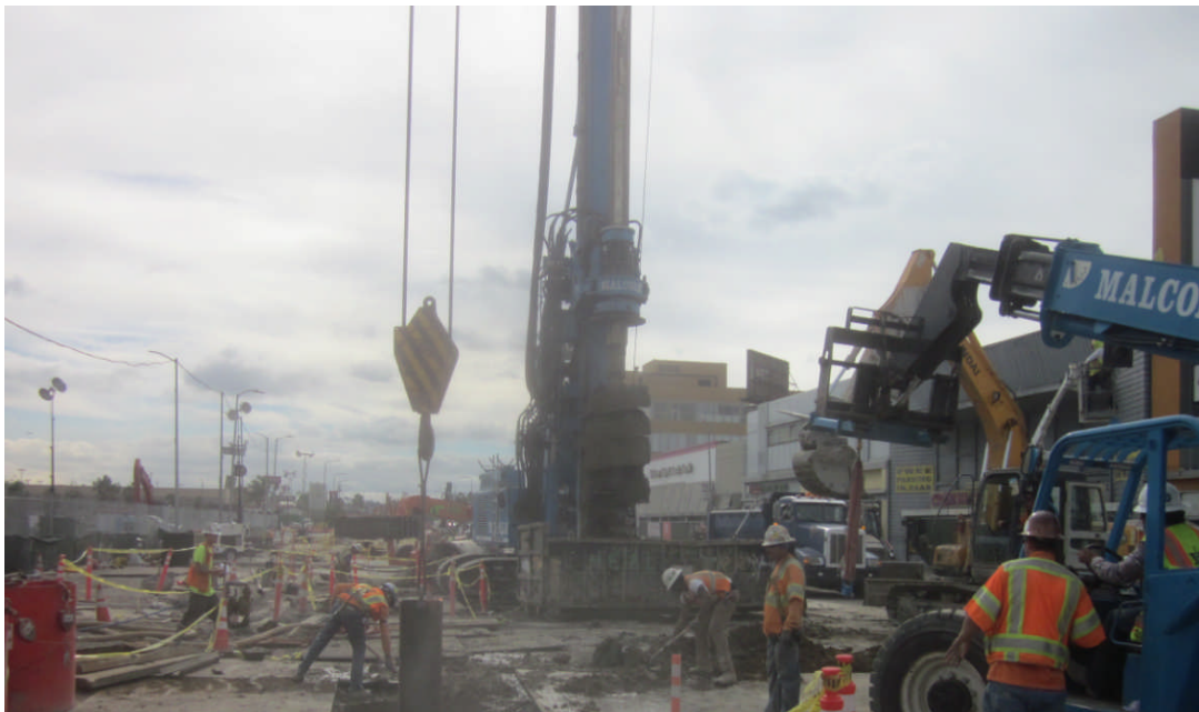
Setting Pin Pile on Crenshaw Boulevard.
