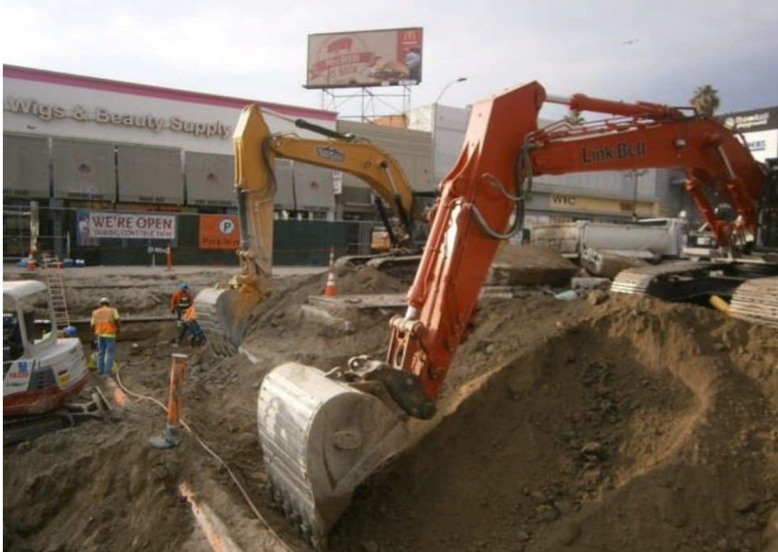
Continued to excavate going north on Crenshaw Boulevard.
