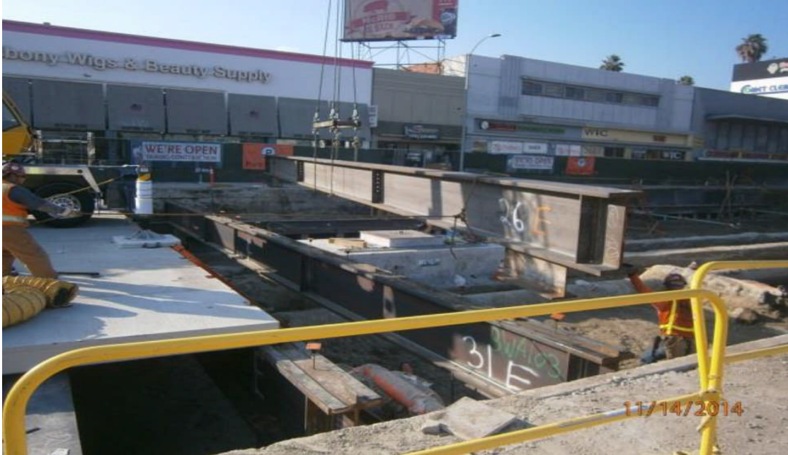
Placing deck beams 25 and 26.
