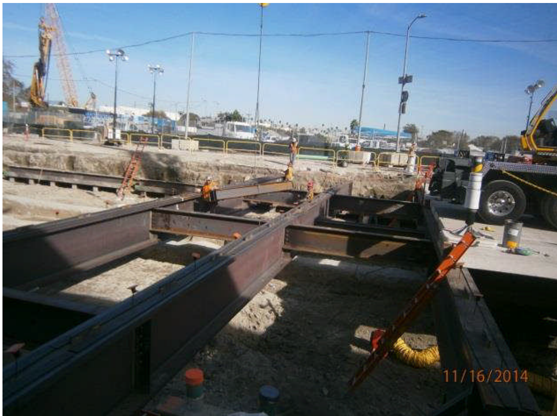
Placing bracing beams for beams 34 and 35.
