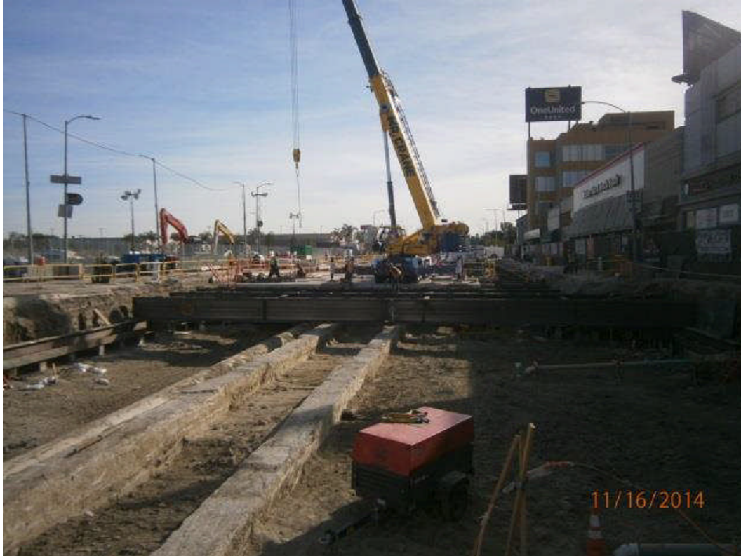
Placing deck beam #34, 35,36 and 37.
