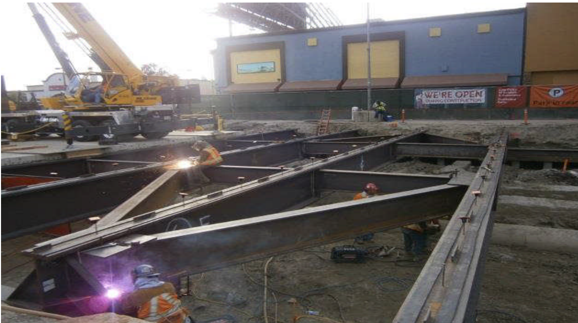
Continue to weld beams on the south side of station.
