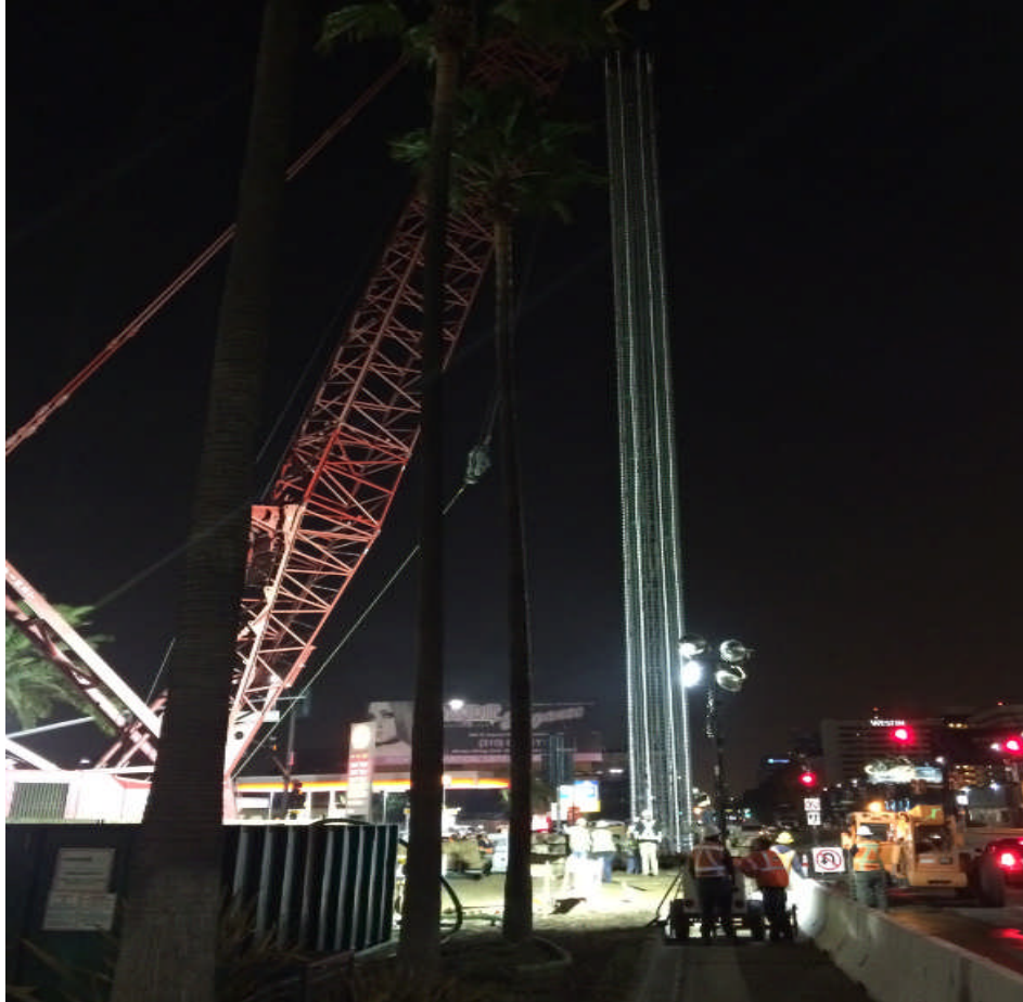
Aviation/Century Aerial Structure CIDH Cage Setting.
