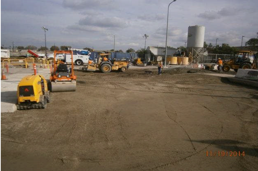
Place base for connecting ramp on Rodeo Place and Crenshaw.
