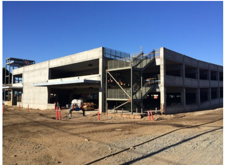
Monrovia Parking Structure Site Overview
