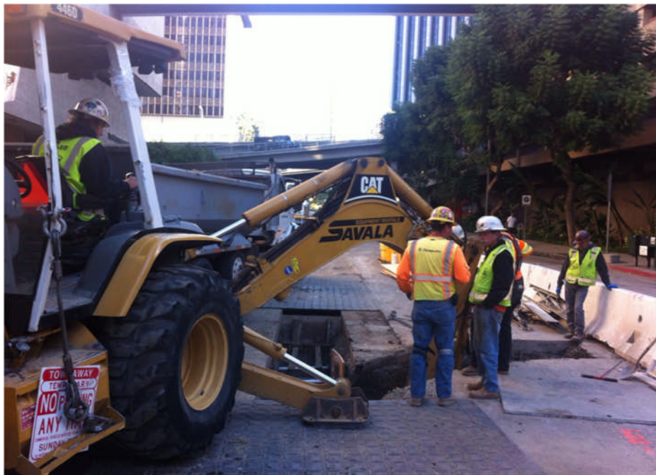
AUR C0981R – Excavation and Shoring at Flower St.
