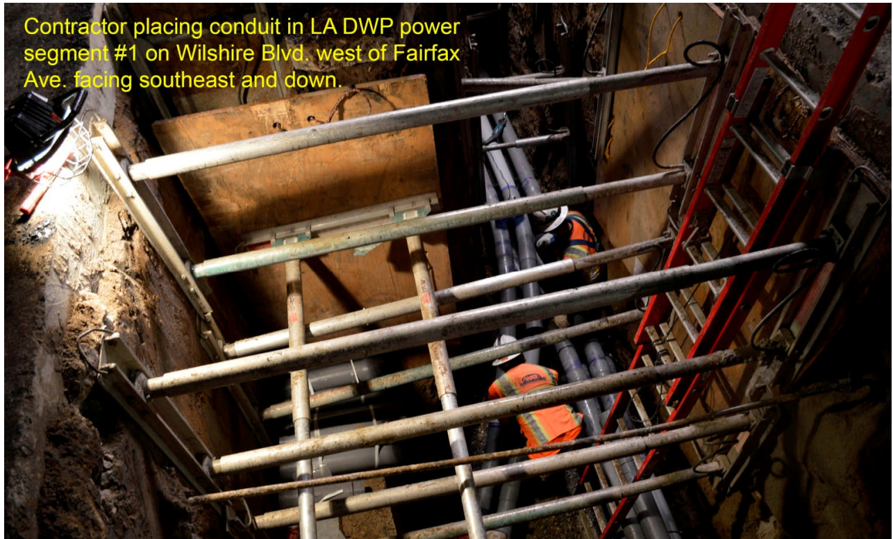
C1055 Contractor Performing Power Relocations on Wilshire Boulevard
