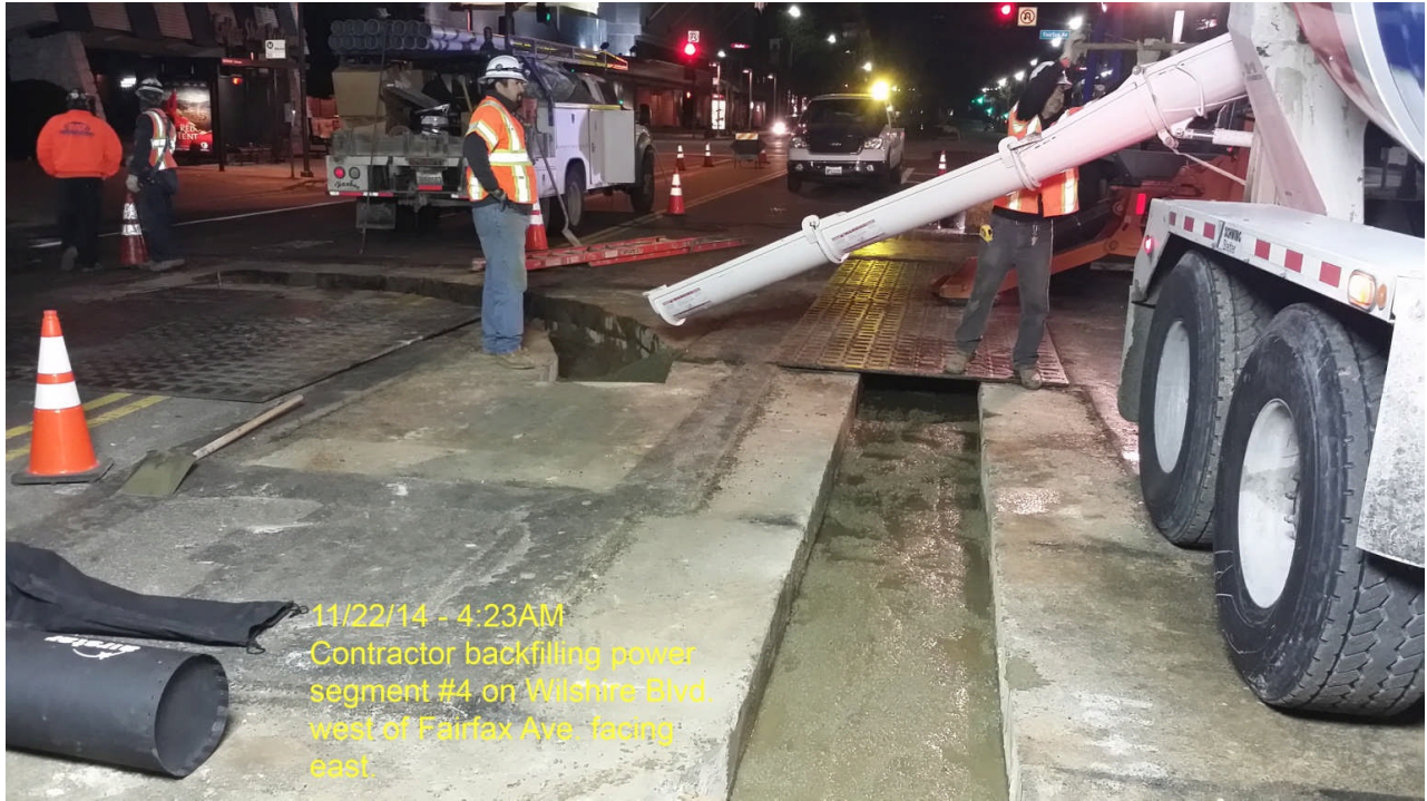
C1055 Contractor Backfilling Power Trench on Fairfax Avenue
