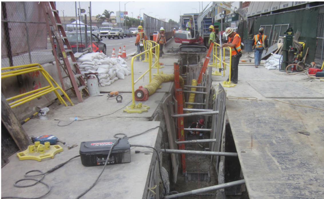
Cutting piles for cap walers.
