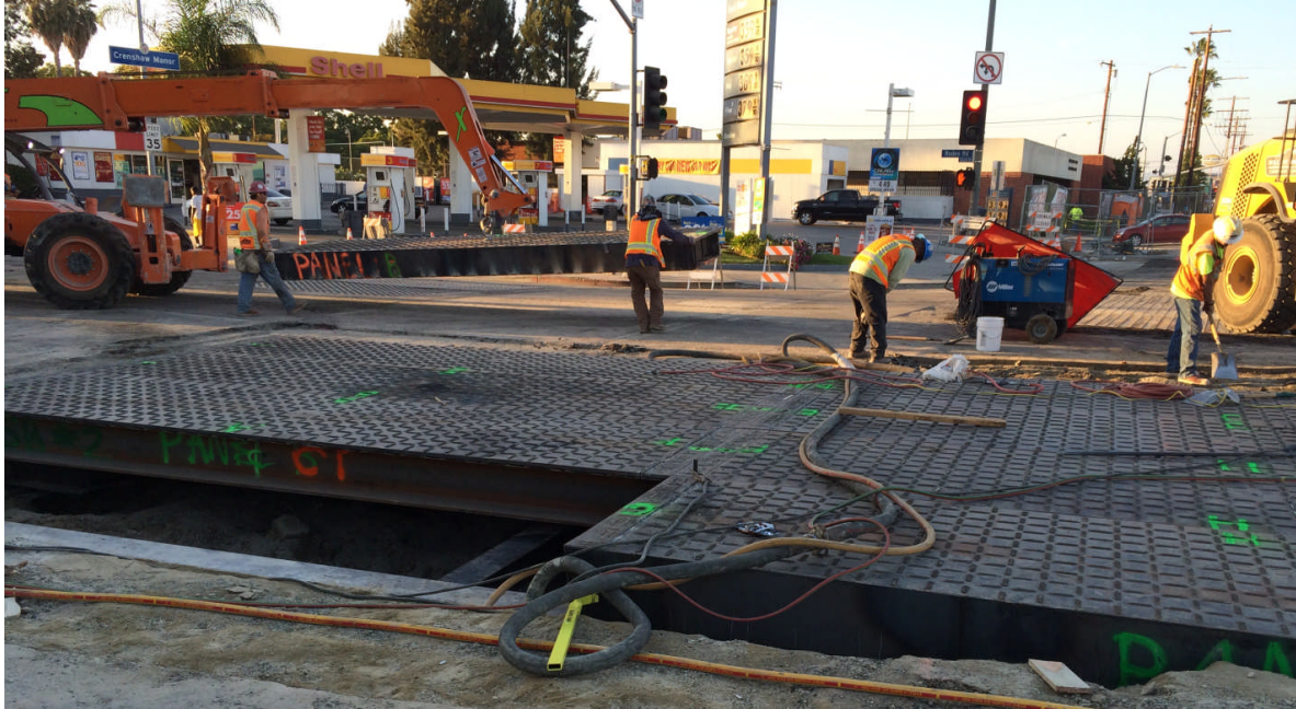
Shoring Top Panels at the Rodeo/Crenshaw Squash Box.
