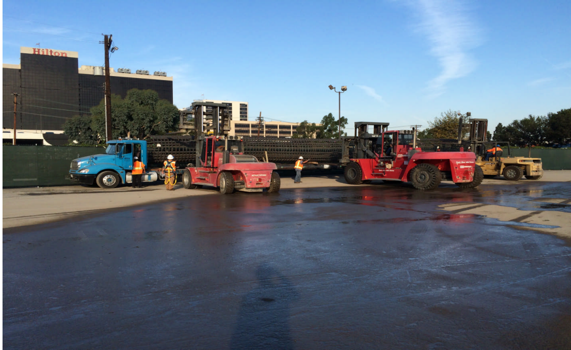
Delivery of rebar cages for the Aviation Century Aerial Structure.
