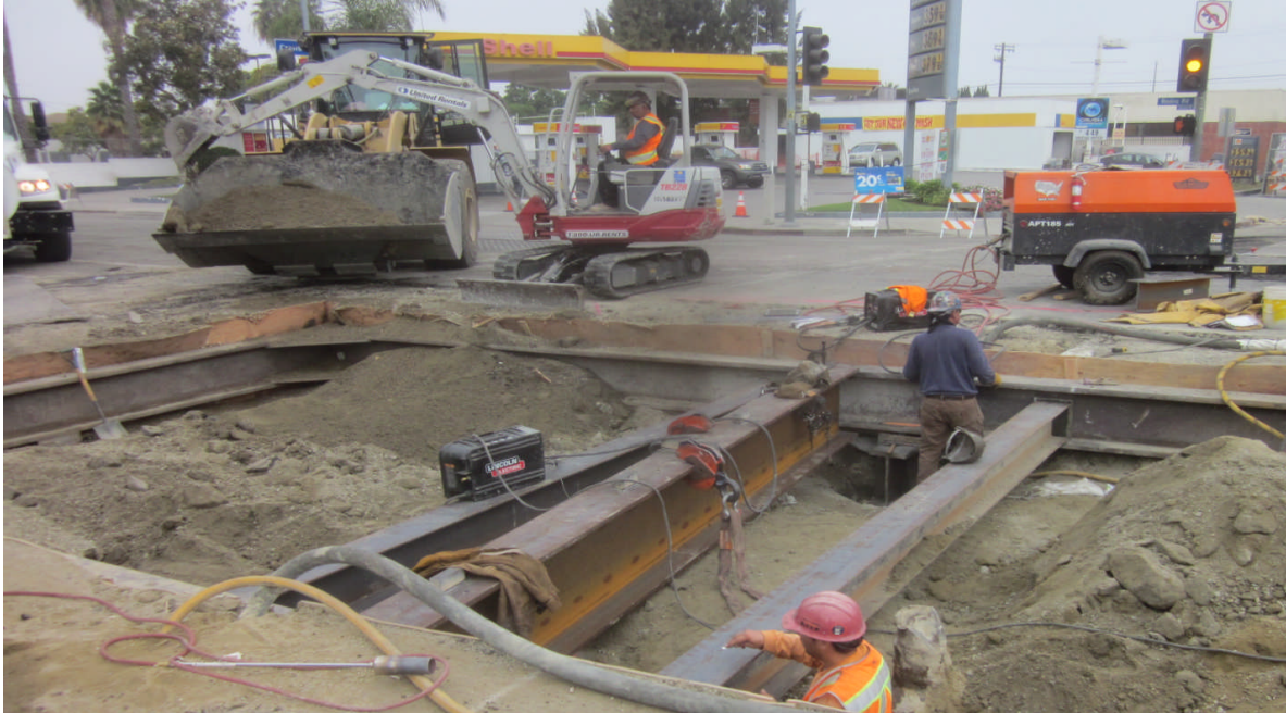
Welding Panel Support Beams in Storm Drain Squash Box.
