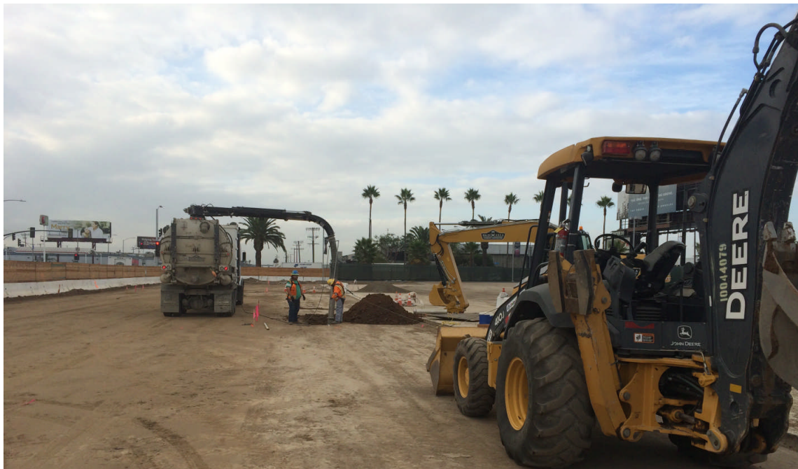
Qwest Fiber Optic Line Potholing.
