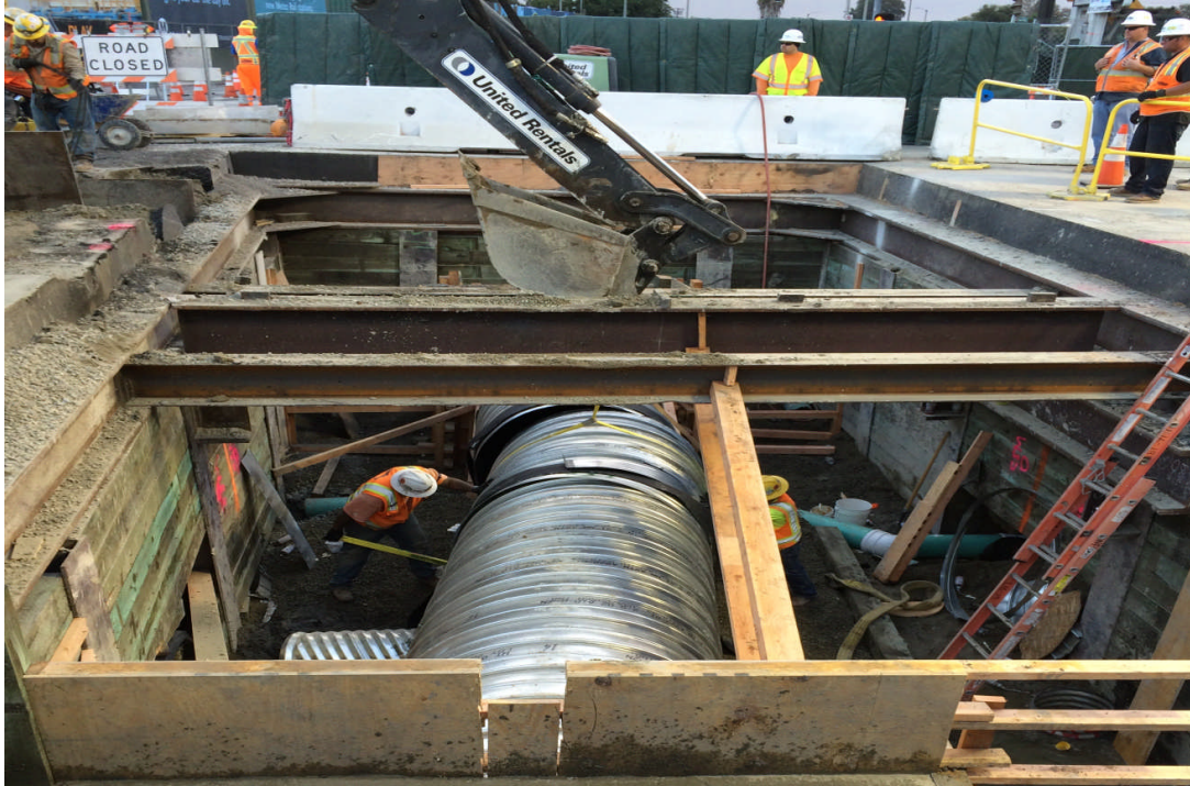
Rodeo/Crenshaw Storm Drain Squash Box.
