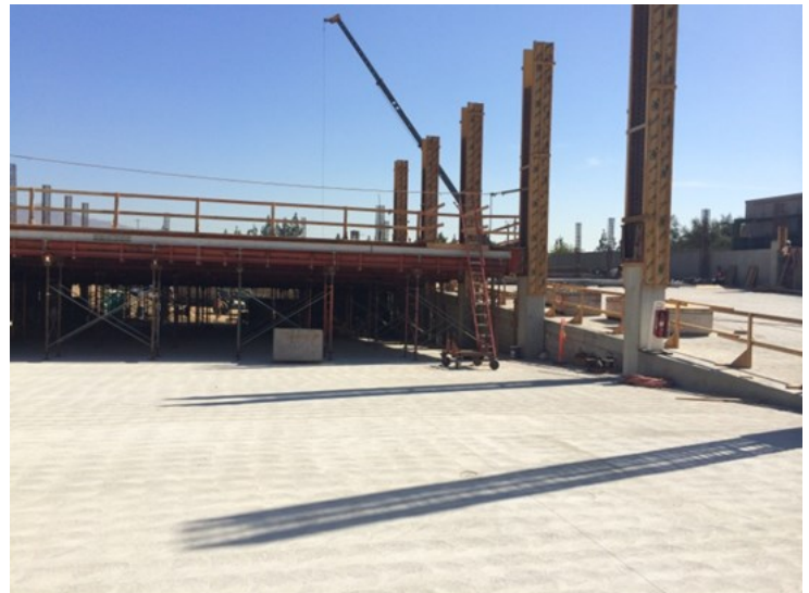
Azusa-Citrus Parking Structure Deck View
