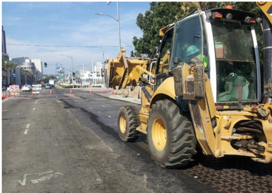
AUR C0981R – Steel Plate and cold mix at edges on Alameda St.
