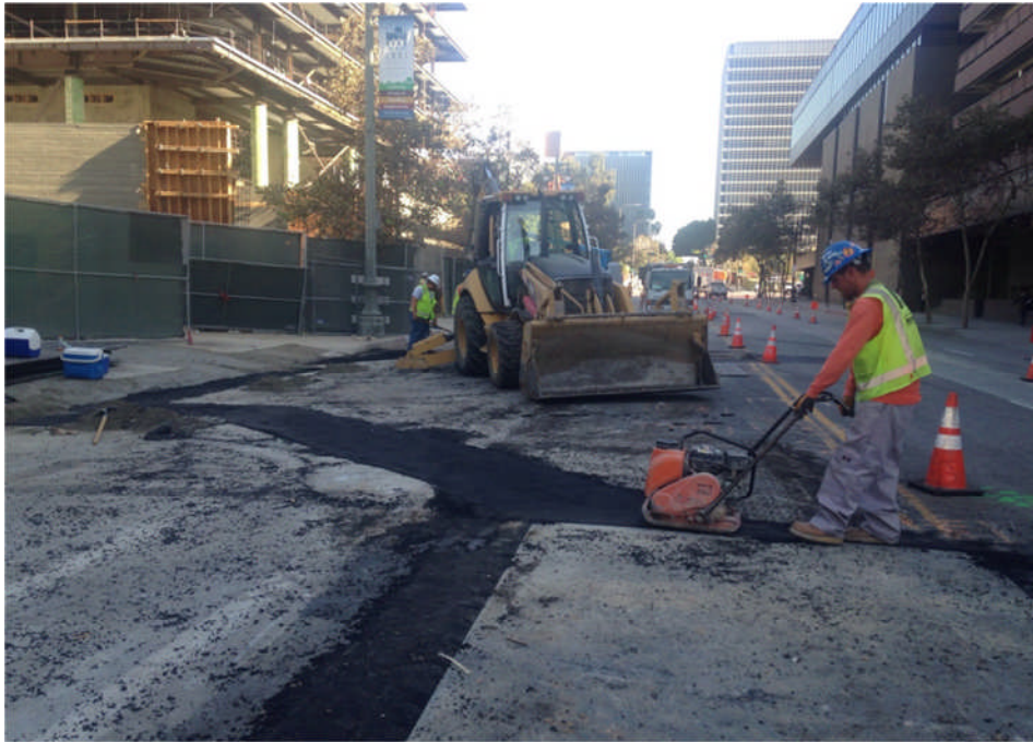
AUR C0981R - Compacting coldmix with a vibra plate at Broadway St.
