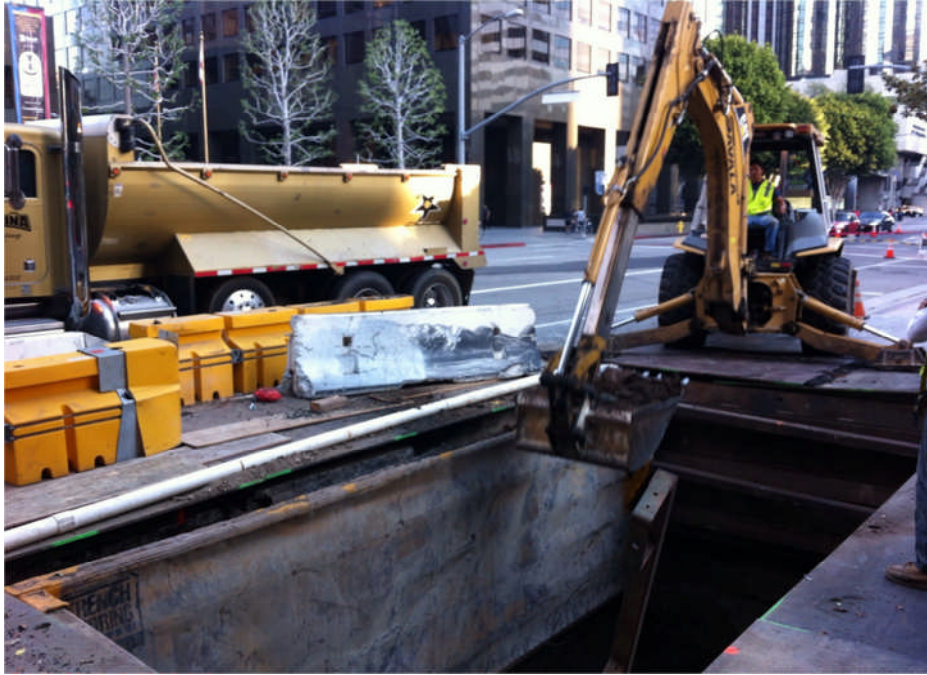
AUR C0981R – Vault excavation on Flower St.
