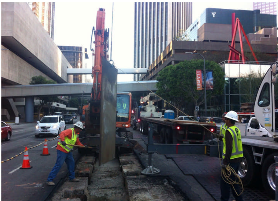
AUR C0981R – Removing metal sheets on Flower St.
