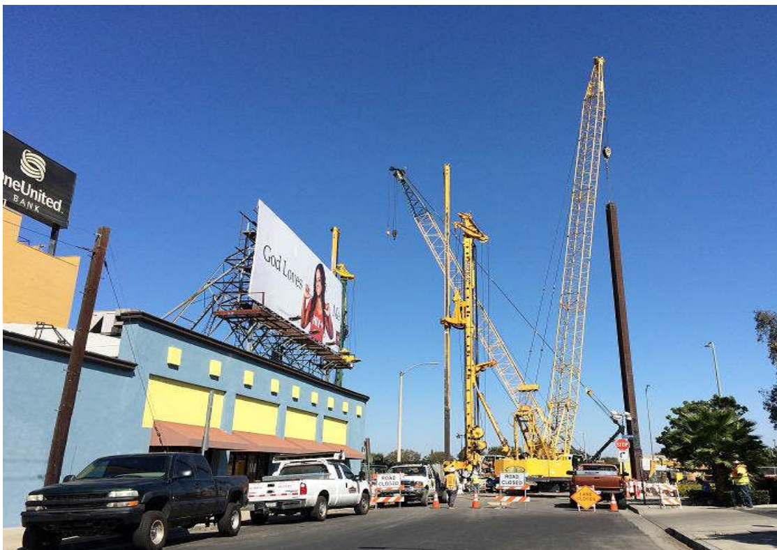
CSM at Expo South Headwall Panel S2 Double Beam.
