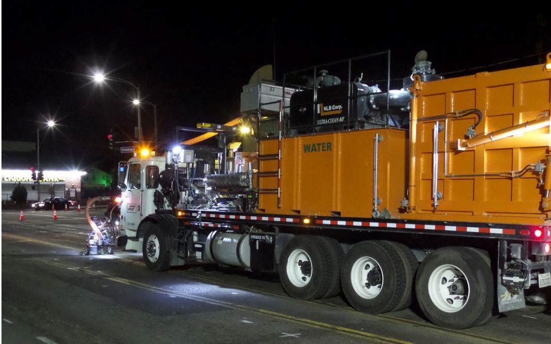
Removing striping by water jetting on Crenshaw.
