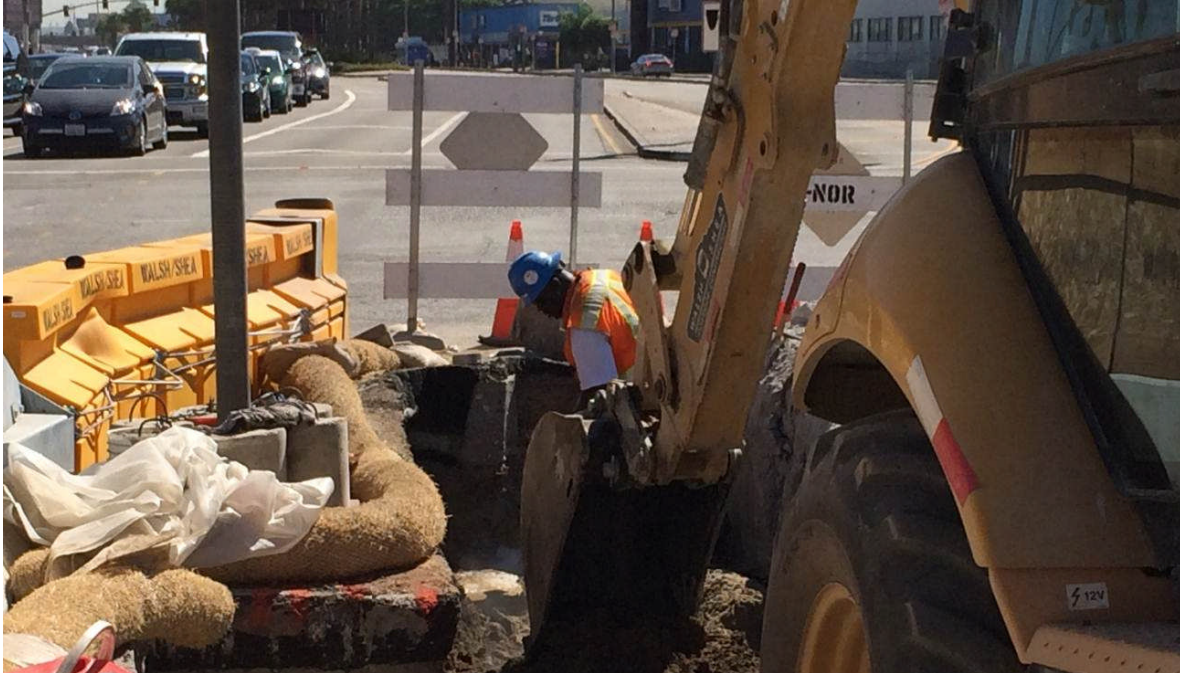
Support of excavation trench on Crenshaw Boulevard (west).
