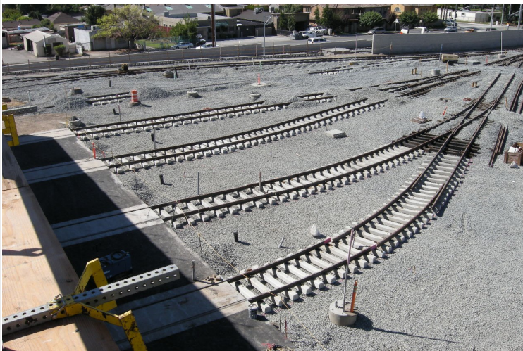
Operations Campus: Shop Lead Track Installations
