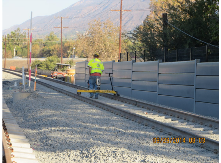
Segment 1: Track Alignment Recording from IFS to Colorado
