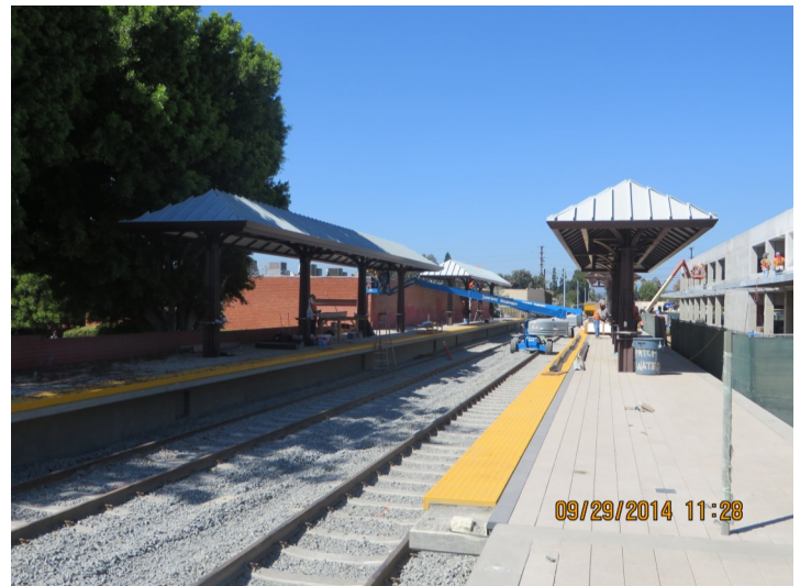
Segment 3: Monrovia Station - Canopy Roof Panel Installation
