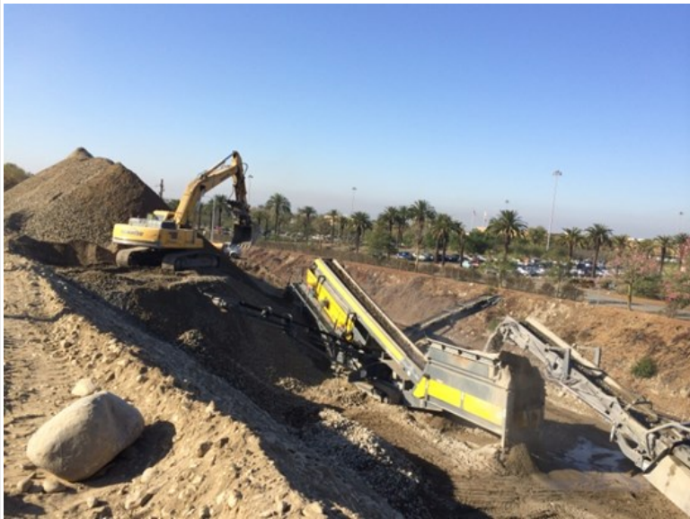
Irwindale Parking Structure Site Excavation
