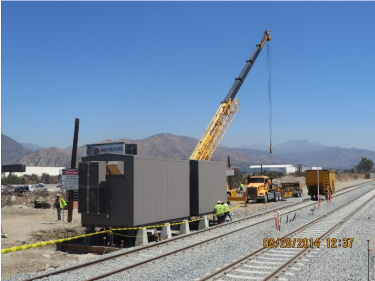
Segment 4: Irwindale Communications Bungalow Installation
