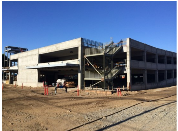
Monrovia Parking Structure Site Overview
