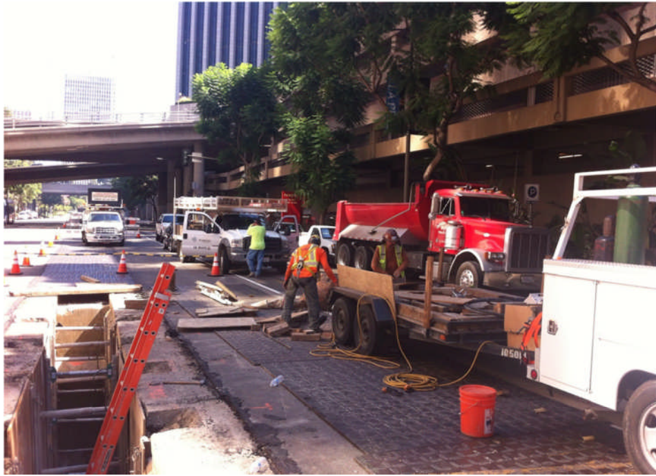
Form and pour encasement for DWP Power on Flower Street
