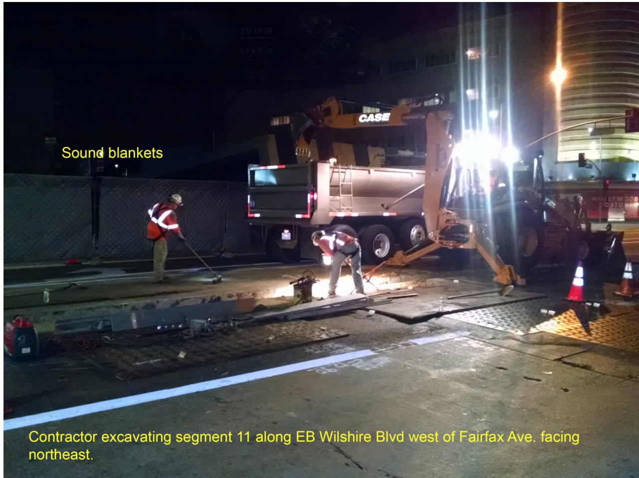
C1055 Contractor Using Sound Blankets to Mitigate Noise in Wilshire/Fairfax Area
