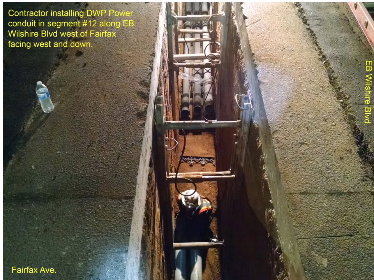
C1055 Contractor Installing Power Conduit at Wilshire/Fairfax Intersection
