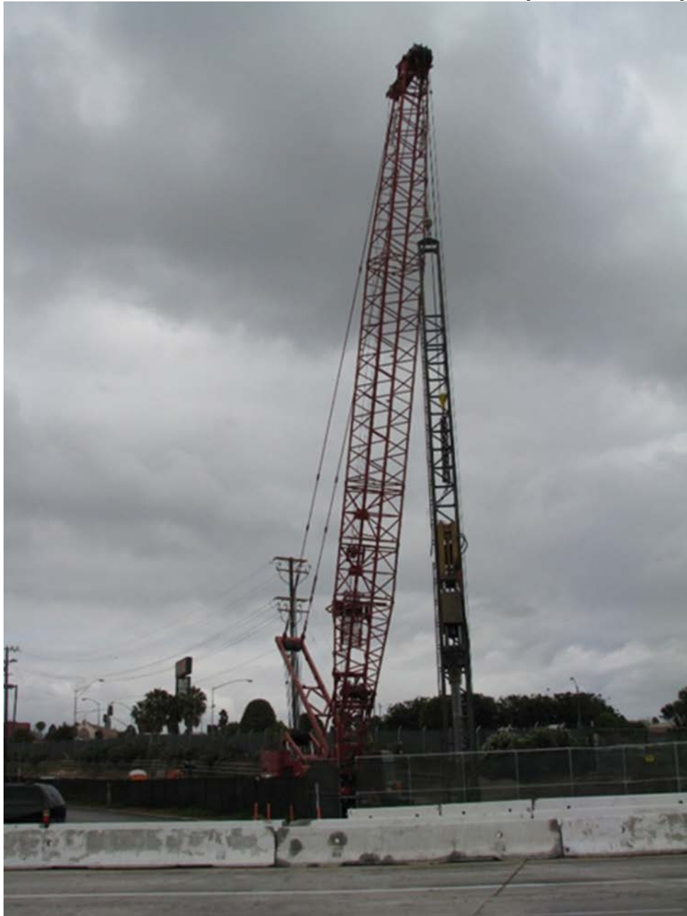
Pile Driving at La Brea Bridge Abutment 2 (East).
