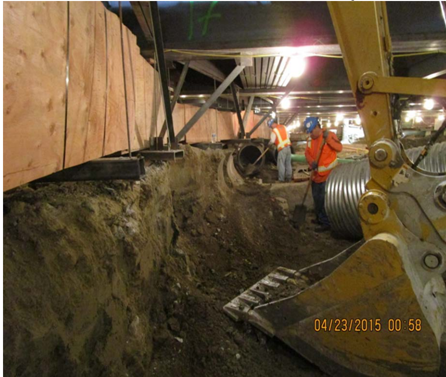
33 inch Storm Drain Replacement and Utility Hanging at MLK.
