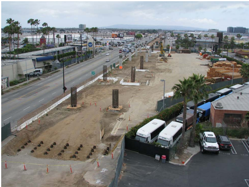
North of Century - Overall View Aviation/Century Bridge (Abutment 10 on the Left).
