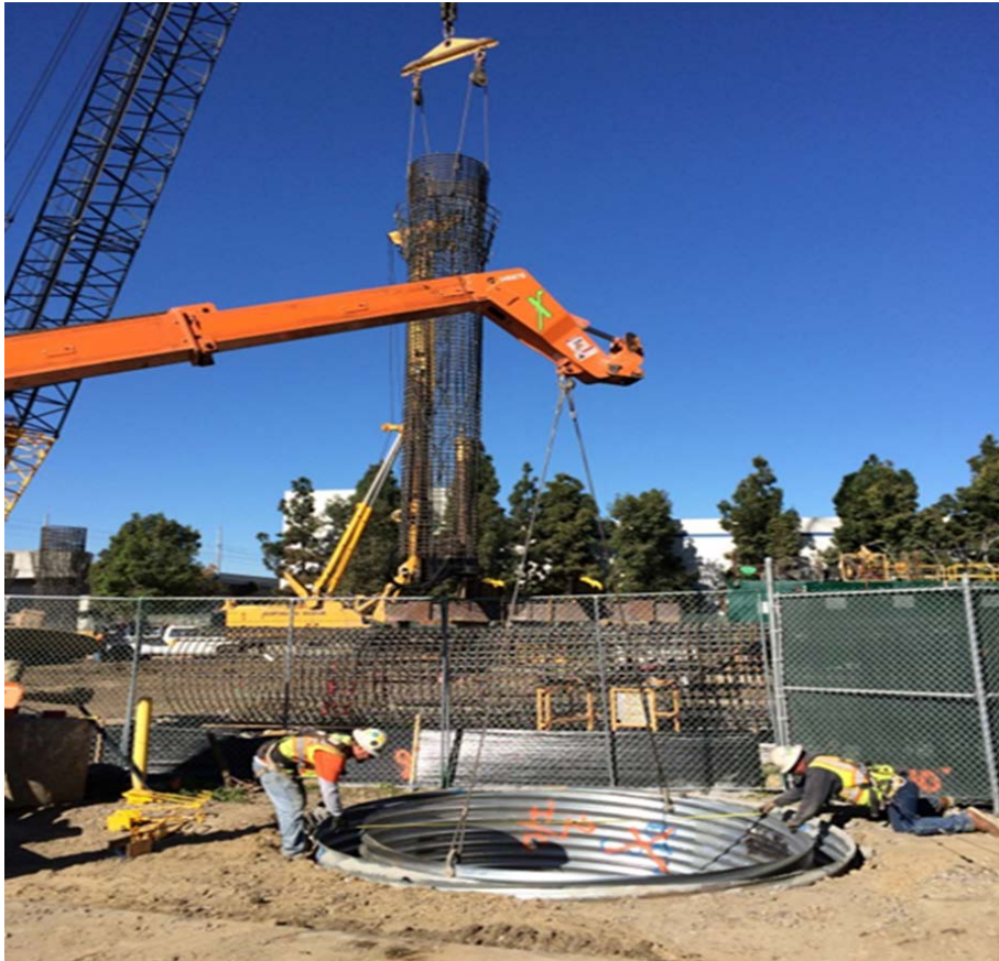
Green Line Bent 2 Isolation Casing.
