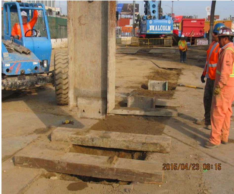
Pile Installation and Drilling at Vernon Station.
