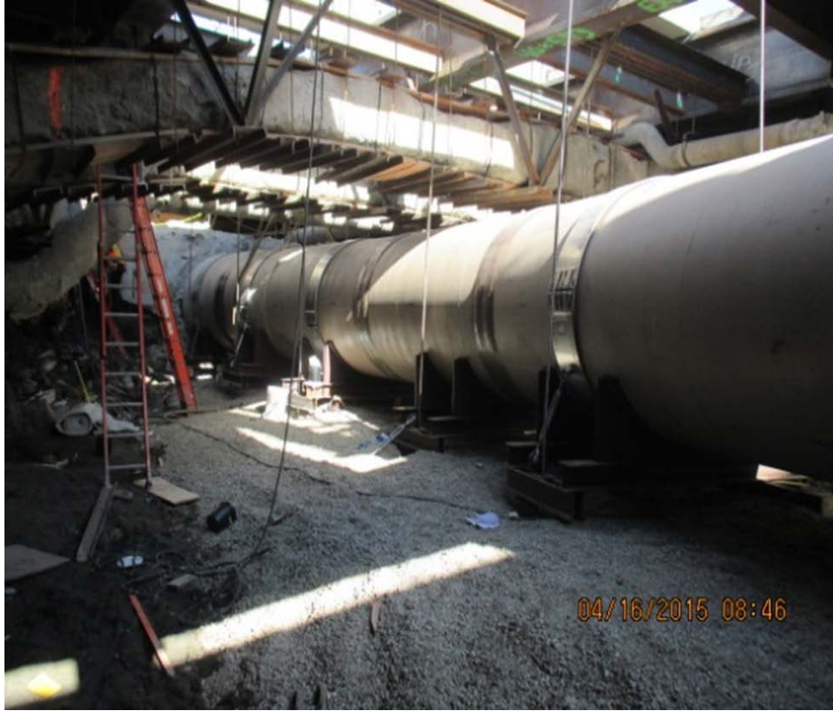
66" Sanitary Sewer Hobas Pipe Installed at Expo Station.
