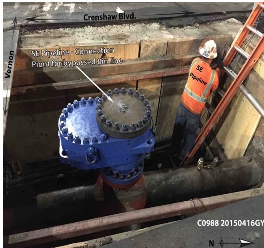
Completed Gas Line Relocation at Vernon.
