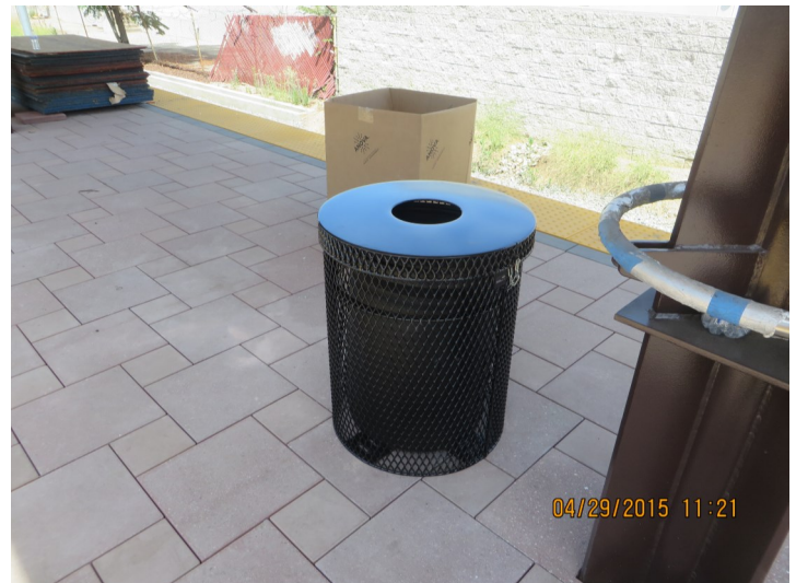
Segment 3: Duarte Station - Trash Cans Installed
