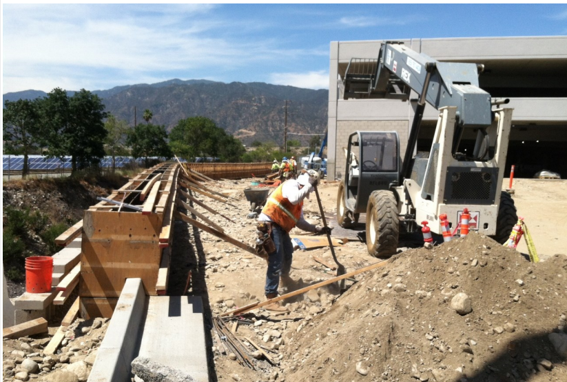
Irwindale Parking Structure Site Work
