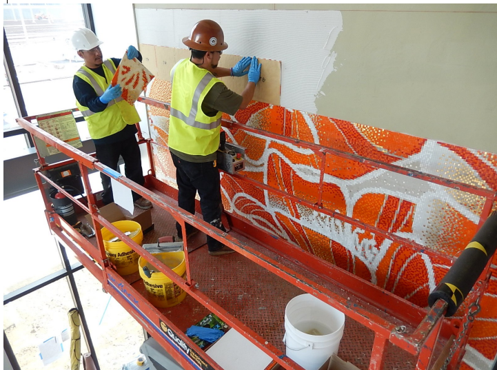
Operations Campus: Work on Lobby Art Wall
