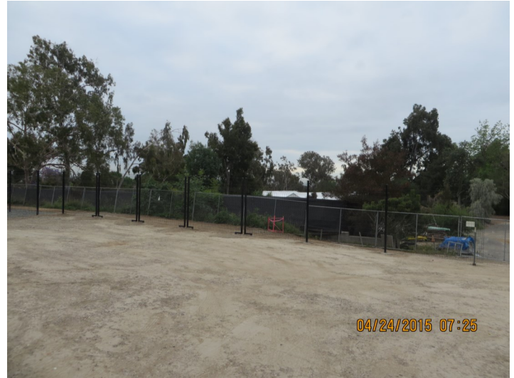
Segment 1: Baldwin TPSS Wire Mesh Fence
