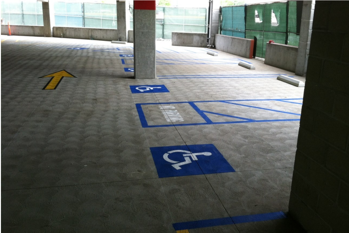
Arcadia Parking Structure Striping
