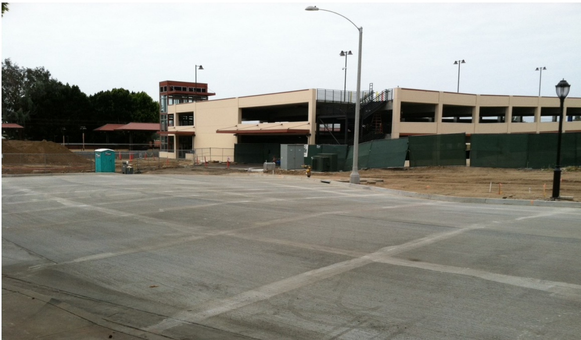
Monrovia Parking Structure Site Overview
