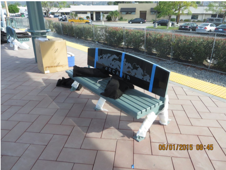
Segment 2: Arcadia Station - Bench Installation
