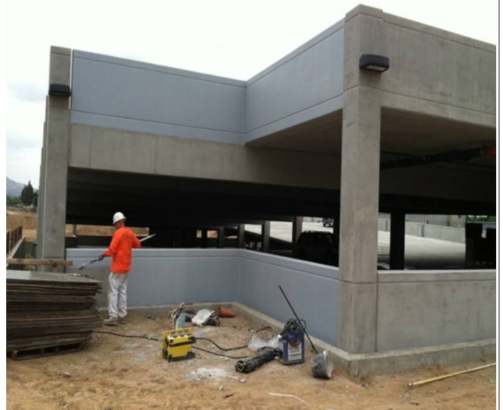
Azusa-Citrus Parking Structure Paint Work
