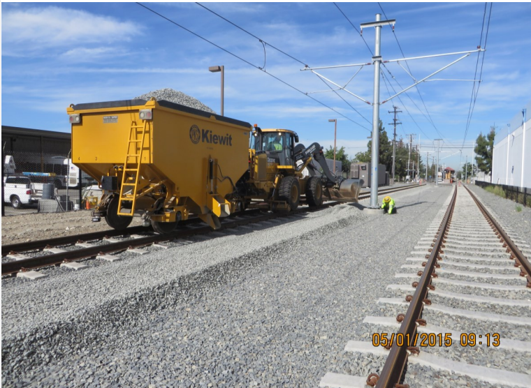
Segment 3: Walkway Ballast Placement
