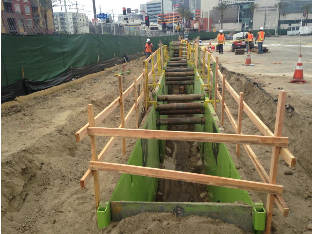
C0980 Contract – Storm Drain at Mangrove yard
