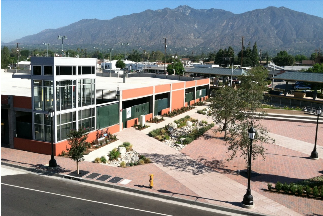
Arcadia Parking Structure Site Overview
