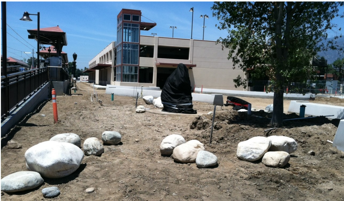
Monrovia Parking Structure Site Overview
