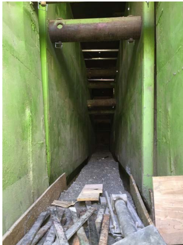
1 st /Rose – Stripping Encasement
