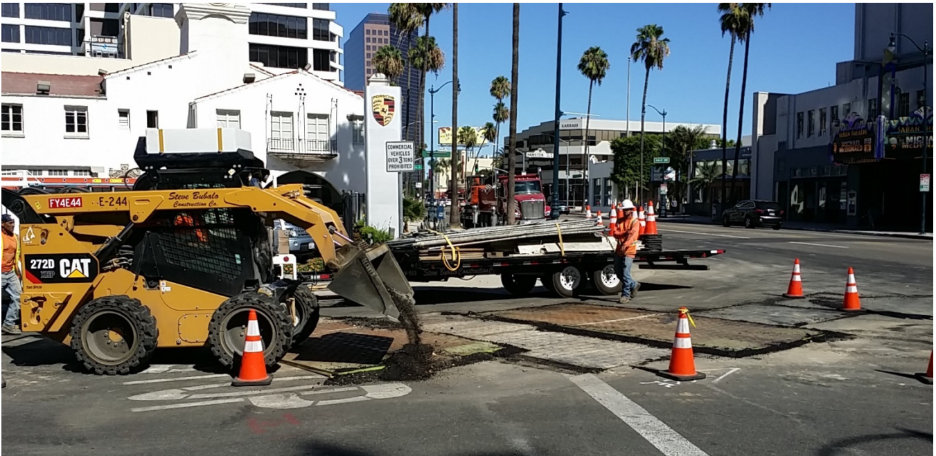
C1056 AUR Contractor Placing Cold Mix Asphalt on Trench Plates
