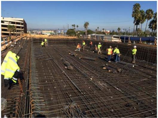
AVIATION/CENTURY – Steel placement of interior stem reinforcement in span 6
