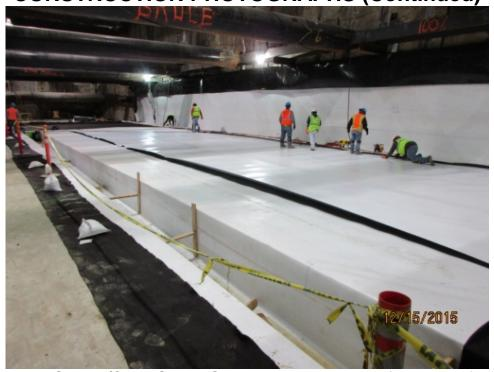
**EXPOSITION/CRENSHAW STATION** – Installation of waterproofing in the south end of station box
