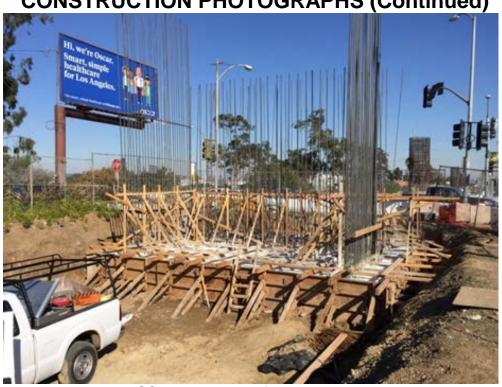
I-405 UNDERPASS - Abutment 1 footing concrete pour and curing
