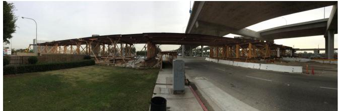
**GREENLINE UNDERPASS**: Falsework construction for superstructure ongoing. Stringers over Imperial have been set.
