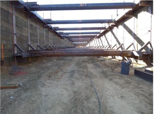
**UG1** - Crews working on tier 2 walers and struts, installing treated wood lagging and removing spoils to haul off-site.
