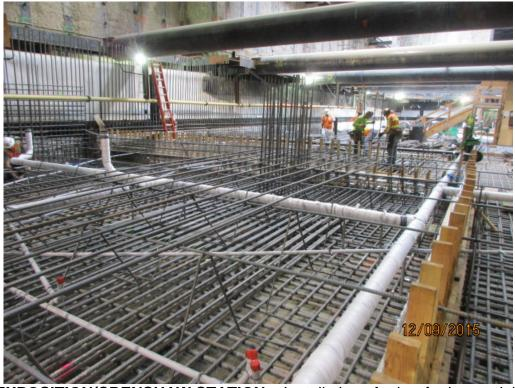
**EXPOSITION/CRENSHAW STATION** – Installation of rebar for invert slab
