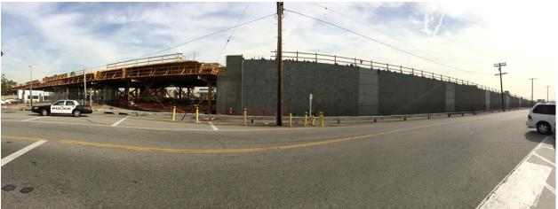
**MSE (Wall 3, 60L&R):** Precast panel erection, placement of soil reinforcement, backfilling and compaction testing complete as of 12/14/15.
