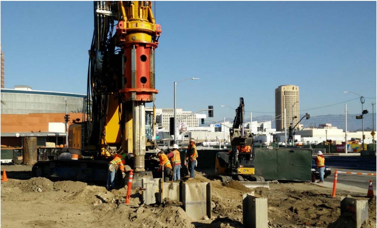
1 st /Central Pile Installation
