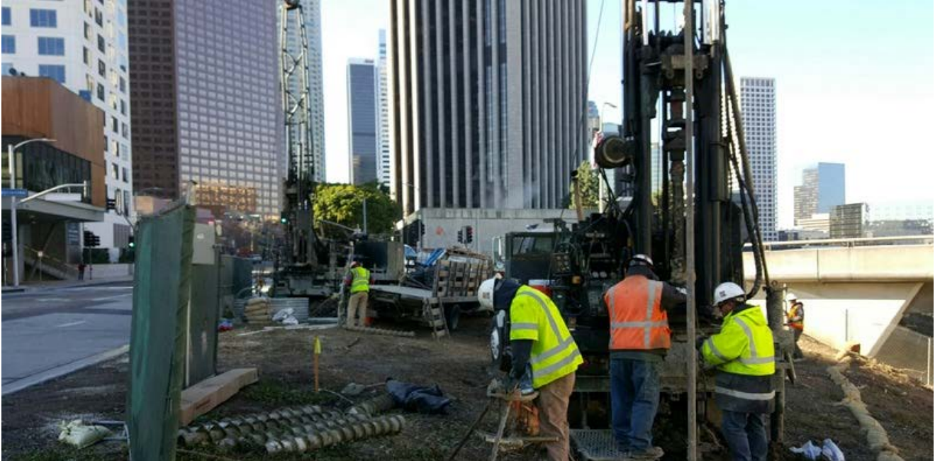
Installing Inclinometer at 2 nd /Hope
