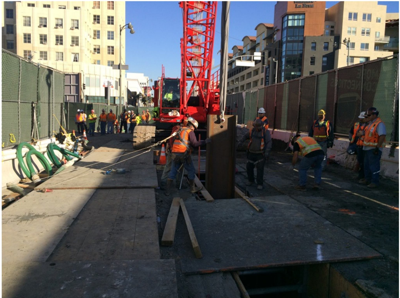
C1045 Contractor Installing the First Wilshire/La Brea Station Pile
