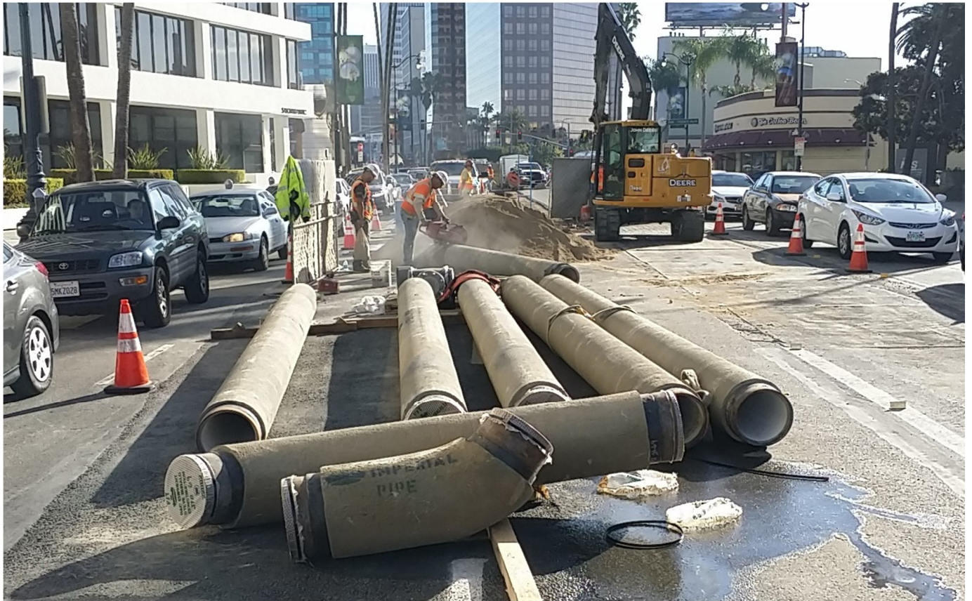
C1056 Contractor Fabricating Water Pipe Prior to Installation
