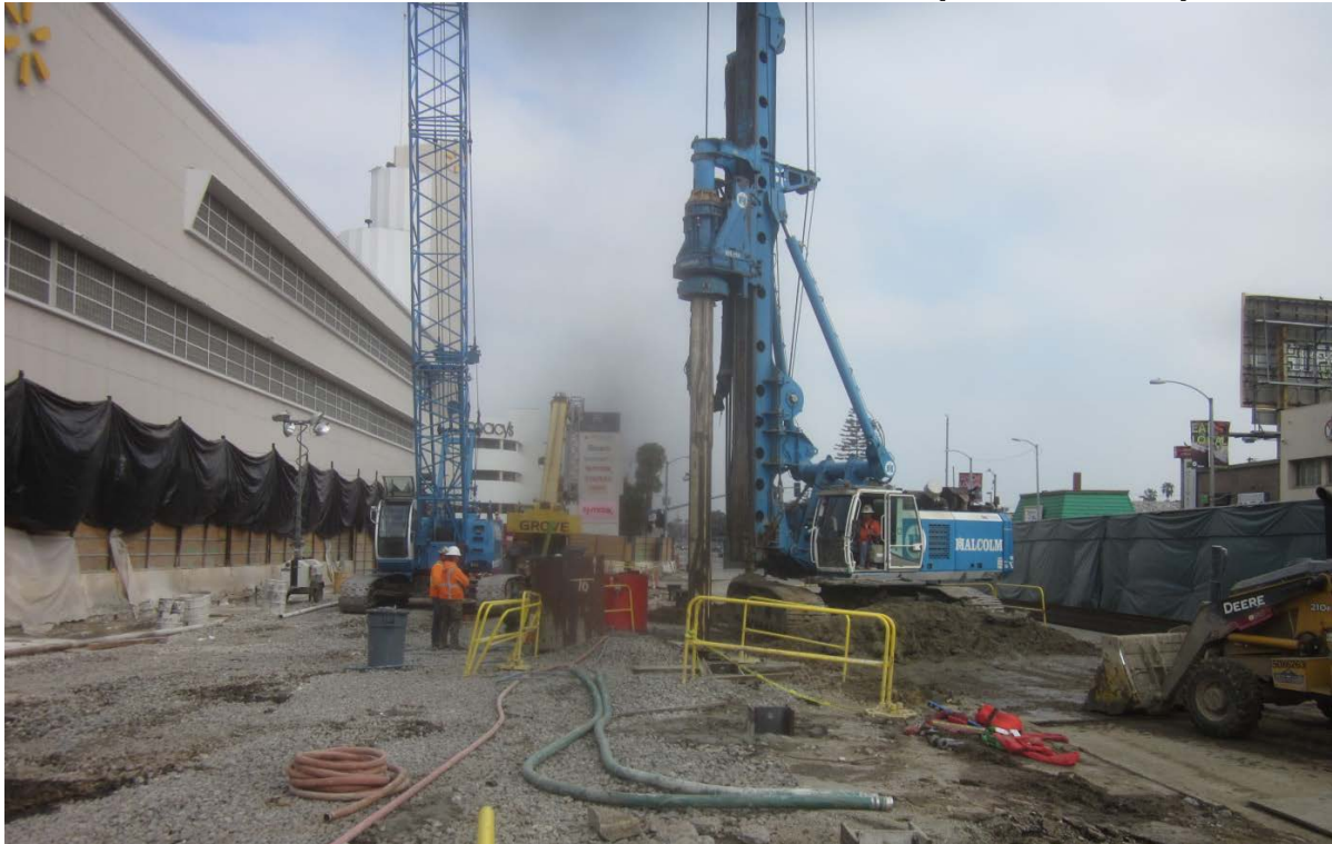
Drilling Pin Piles for Excavation Support at MLK Station.
