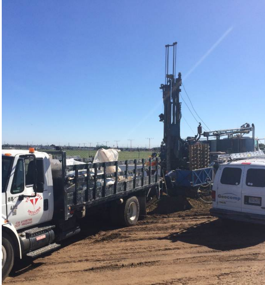
UG#1 Inclinometer Installation at Sta 41+50.
