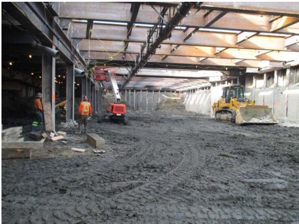
WSSC removing soil from the north end of the Expo Station.
