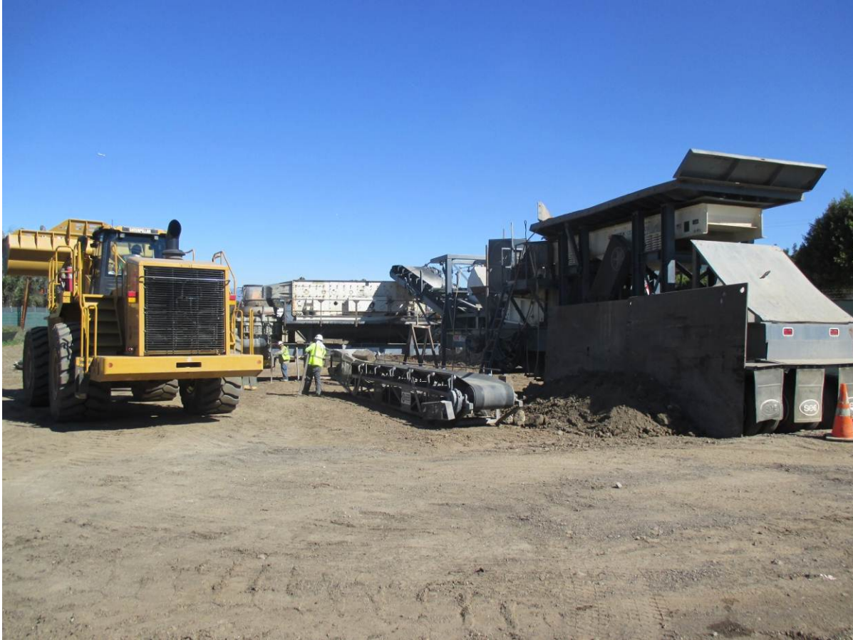
Concrete Recycling Facility (assembling) at La Brea Station.
