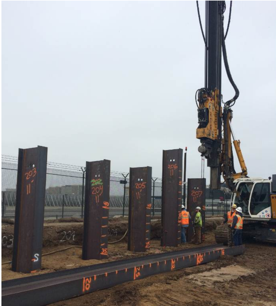
UG#1 Zone 2A Support of Excavation Pile 203 to 207.
