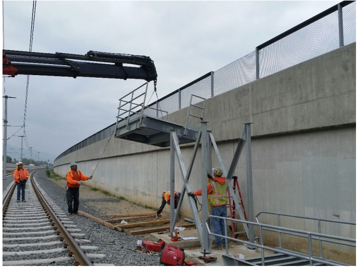
Segment 1: Sierra Madre Villa - Emergency Egress Stair Installation
