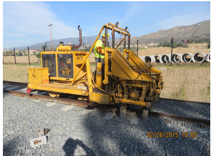
Segment 4: Citrus to Barranca - Track Surfacing
