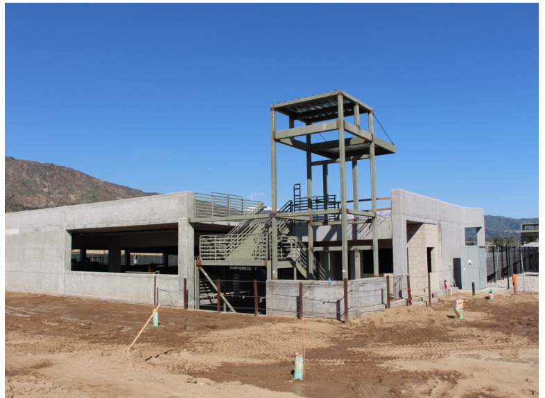
Azusa-Citrus Parking Structure Site Overview
