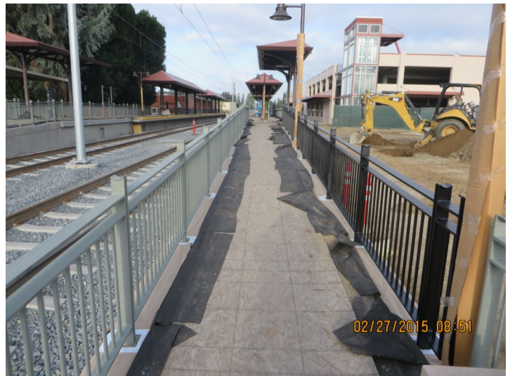
Segment 3: Monrovia Station - Guardrail Painting
