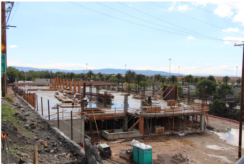
Irwindale Parking Structure Site Overview
