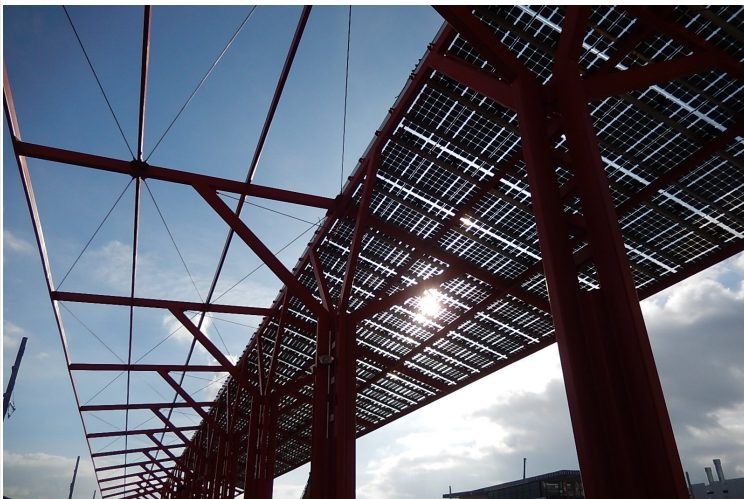
Operations Campus: Solar Panel Installation on the MOW Canopy
