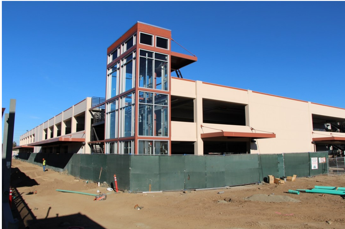
Monrovia Parking Structure Site Overview
