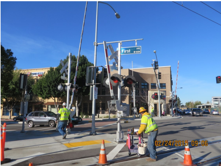
Segment 2: 1st/Santa Clara - Gate Arm Installation and Adjustment
