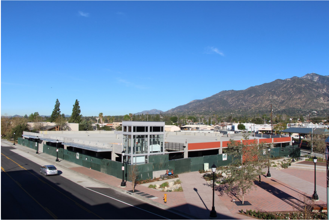
Arcadia Parking Structure Site Overview
