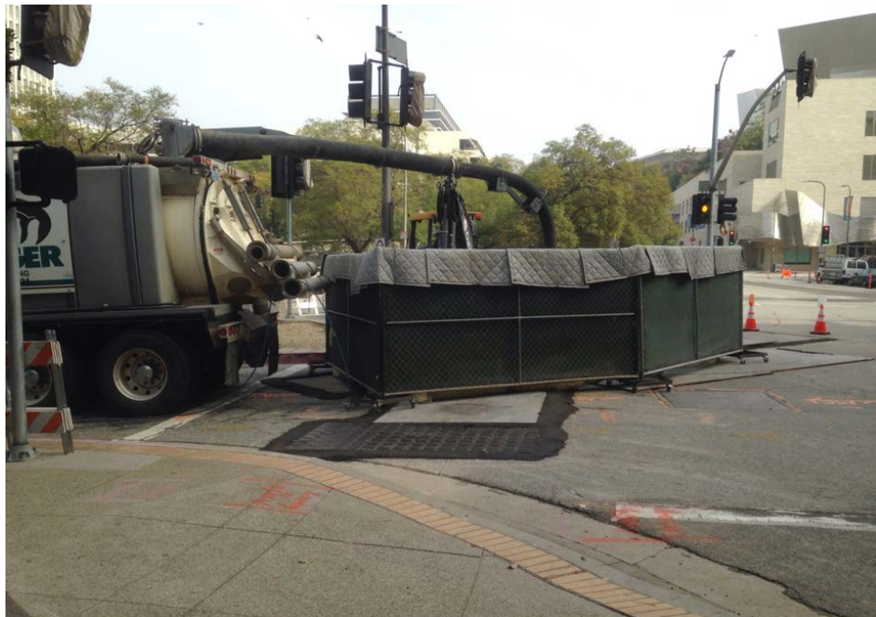
C0980 Contract – Potholing at 2 nd /Hope Sts.
