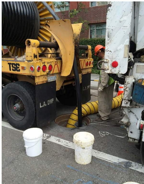
AUR C0981R – DWP Power pulling cable on 1 st /Alameda Sts.
