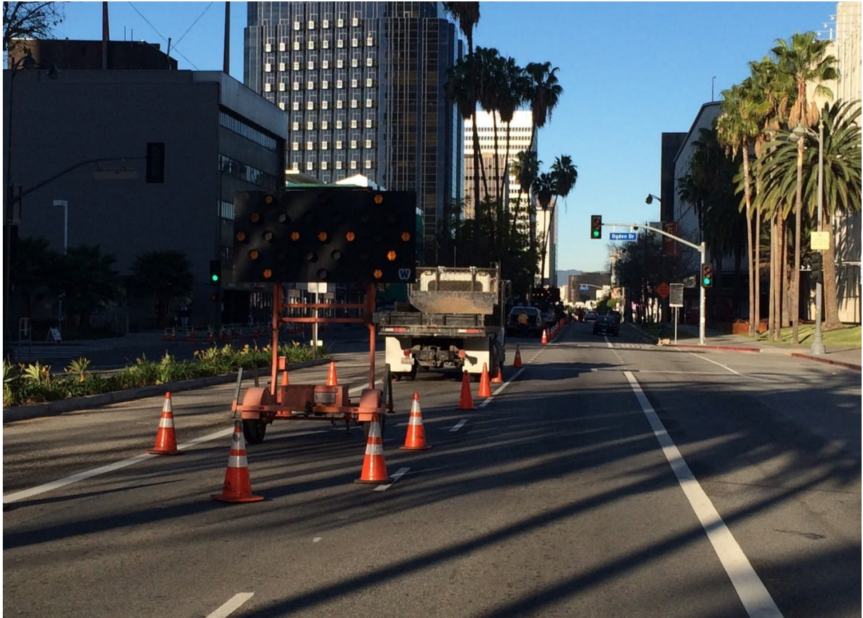
C1055 Contractor Traffic Control West on Wilshire Blvd.
