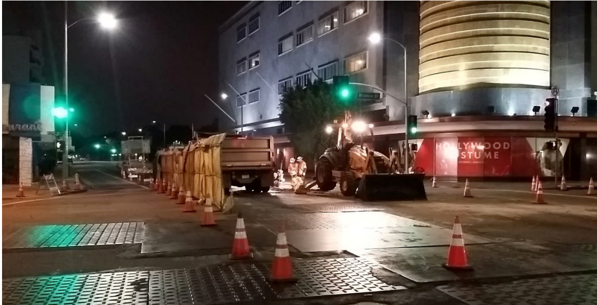
C1055 Contractor Excavating Segment 10 Power Trench at Wilshire and Fairfax
