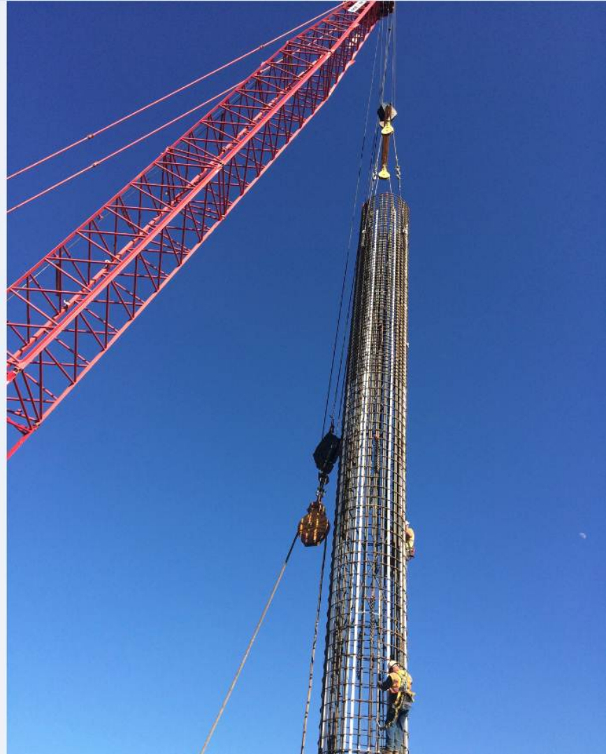
Aviation Century Aerial Structure – CIDH Rebar Cage.
