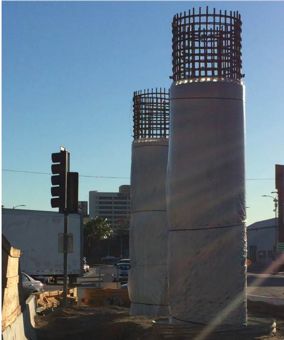
Aviation Century Aerial Structure Visqueen Crapped Curing at Columns.
