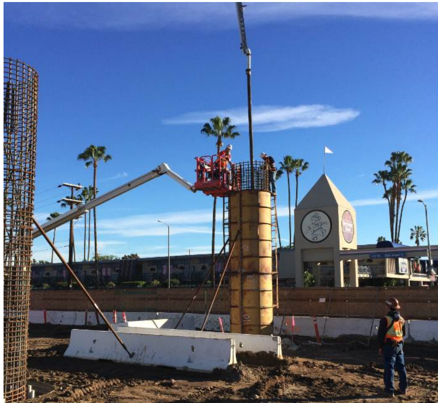
Aviation Century Aerial Structure Column Concrete Placement.
