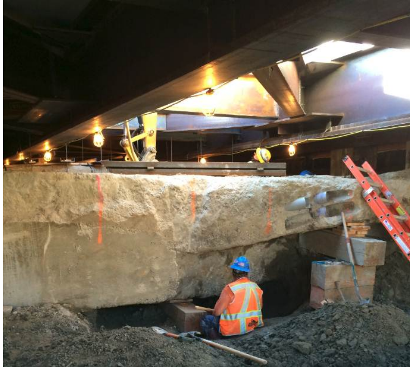
Expo Station Decking Support of Excavation at DWP ductbank.
