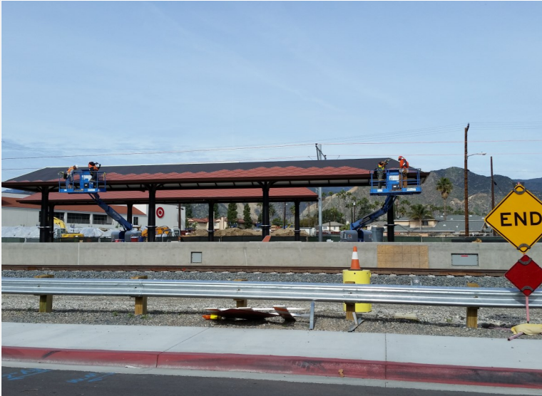
Segment 4: Azusa Downtown Station Progress
