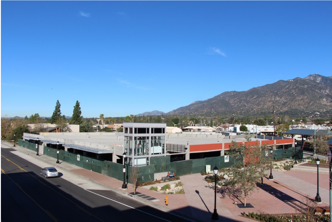
Arcadia Parking Structure Site Overview
