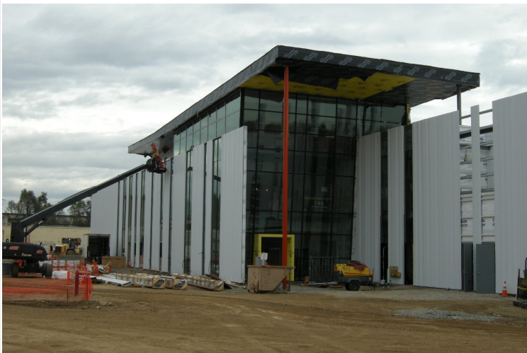
Operations Campus: Glazing at Main Entry nearing completion
