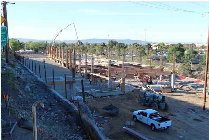
Irwindale Parking Structure Site Overview
