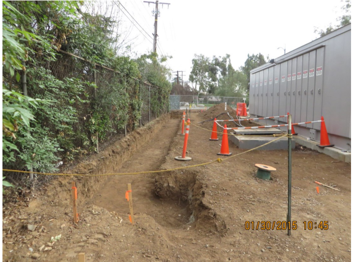
Segment 1: Baldwin TPSS - CMU Wall Excavation
