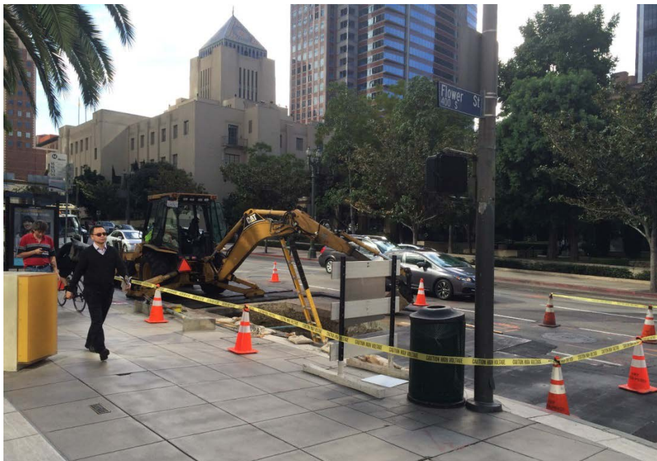
AUR C0981R – DWP Power 3 rd Party Intercept work at Flower St.
