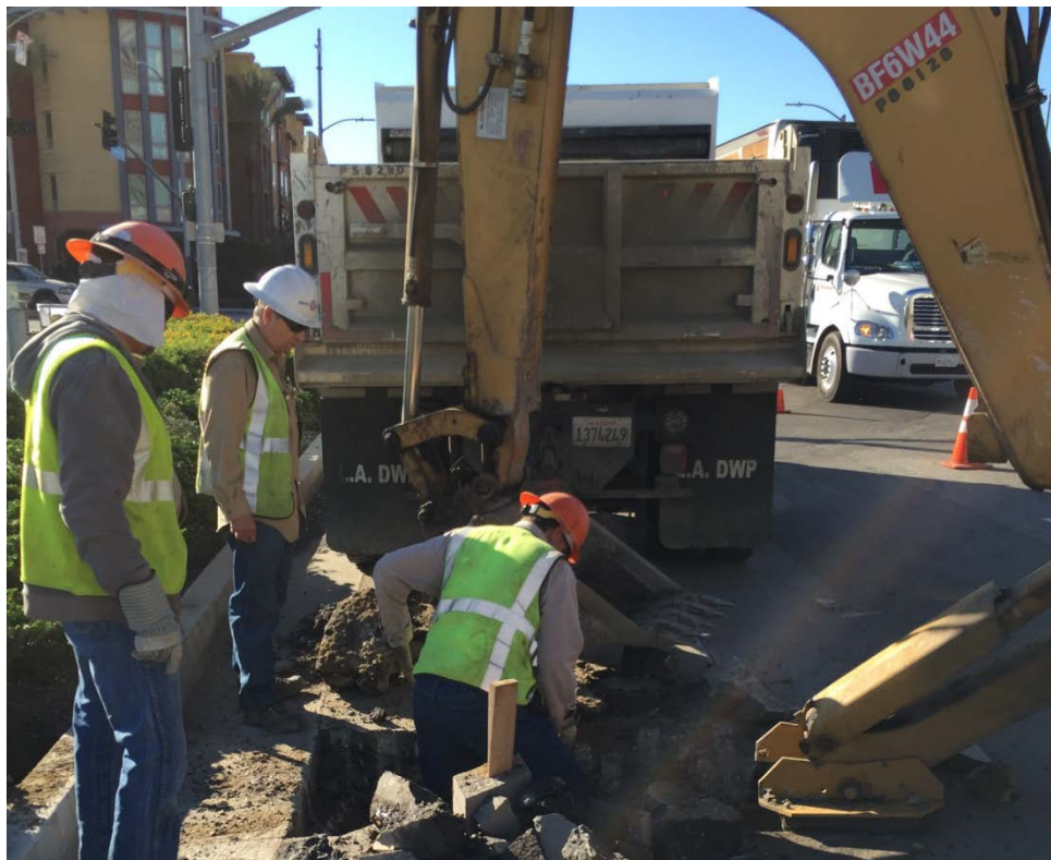
AUR C0981R – DWP Intercept work north of Alameda Street
