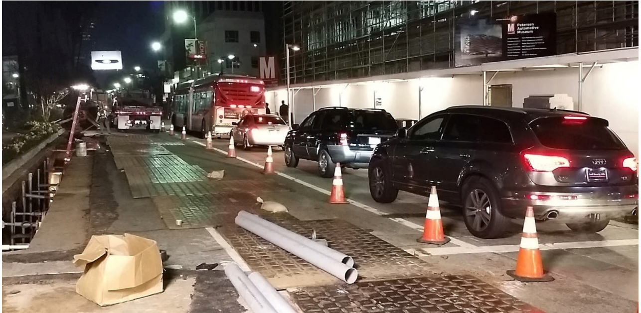
C1055 Contractor Performing Utility Relocations along Wilshire Blvd.
