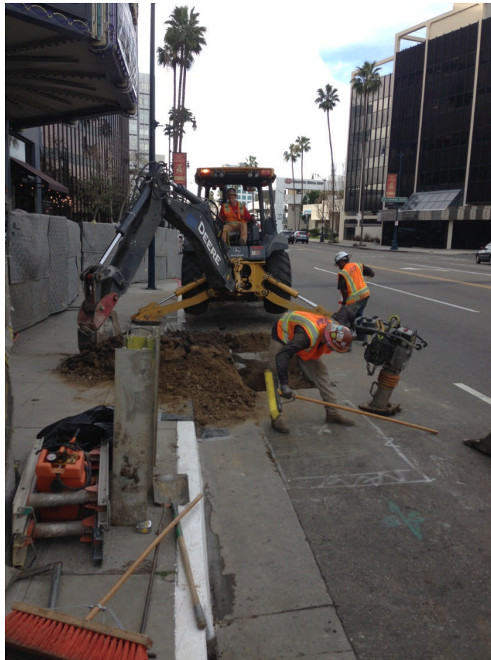
Utility Potholing by VCI at Wilshire/La Cienega
