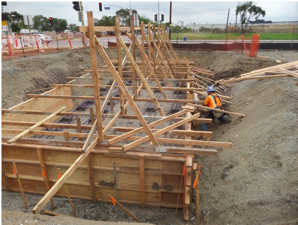
111 TH STREET – Installing form kickers for Abutment #1 footer.
