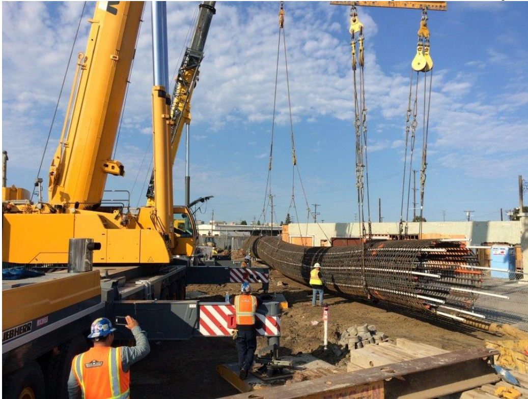
MANCHESTER UNDERPASS – Bent 2 CIDH Rebar Cage Dobot Placement and Debris Removal
