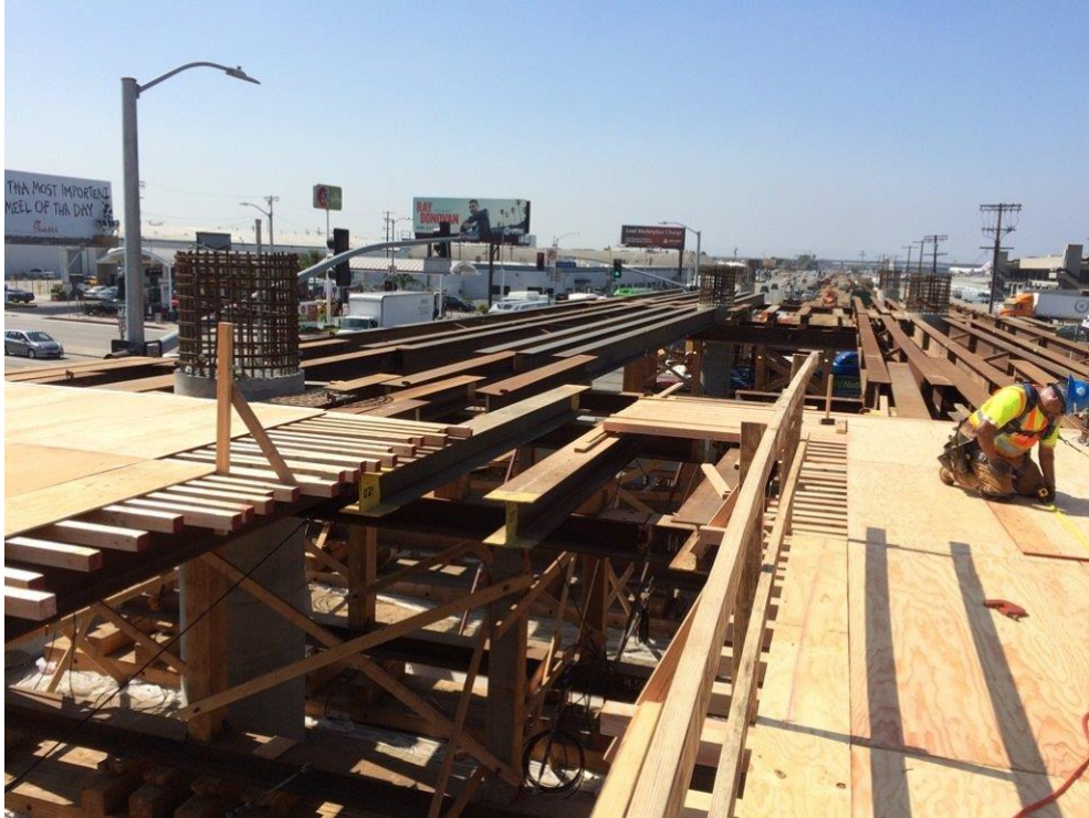
CENTURY/AVIATION – Falsework and rolling soffit
