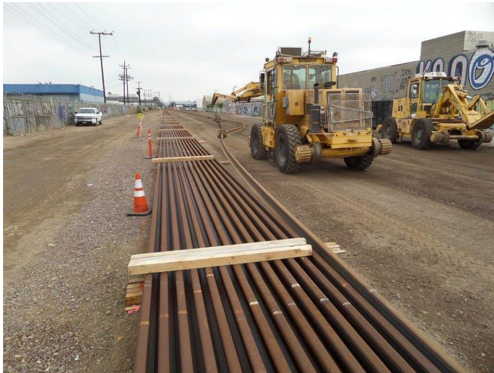
ARBOR VITAE (near Southwestern Yard Site) - Herzog Threading CWR onto Stockpile.
