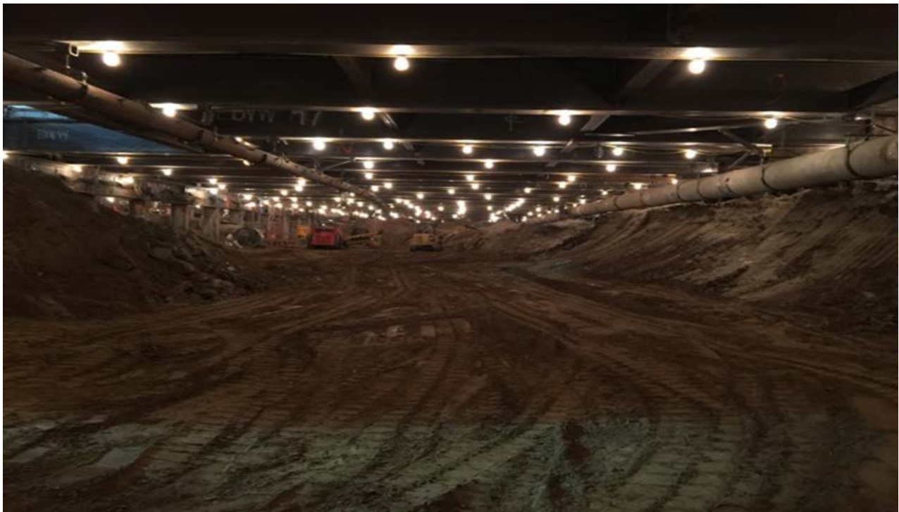
VERNON – Excavation of station box looking south.
