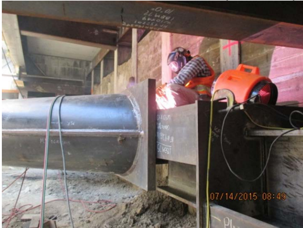
MLK STATION –Welding of northwest corner strut.
