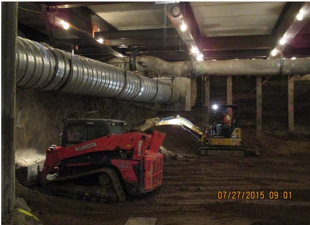
VERNON STATION -On going excavation operations.
