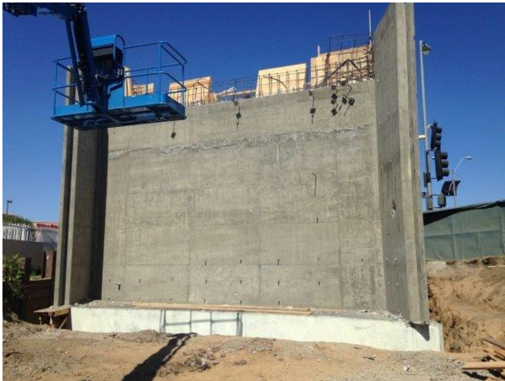
LA BREA – Abutment #1 stripped wall.
