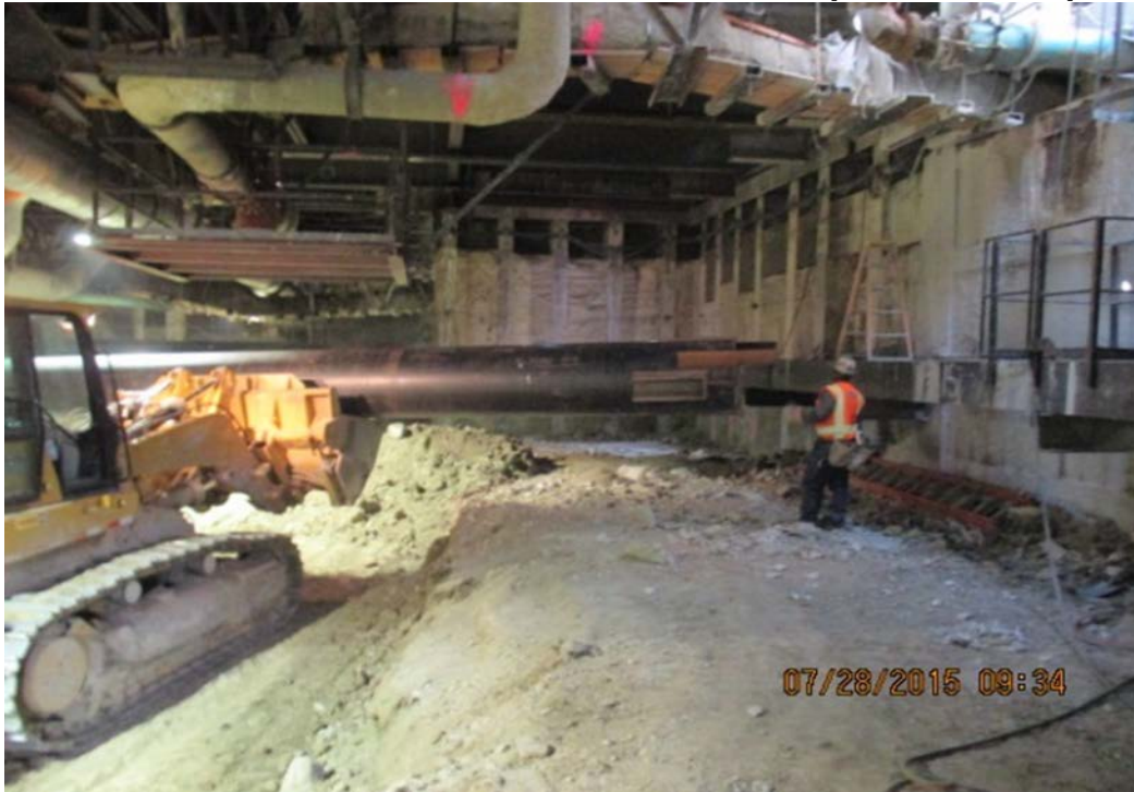
MLK STATION - Struts staged/in-work and excavation operations.
