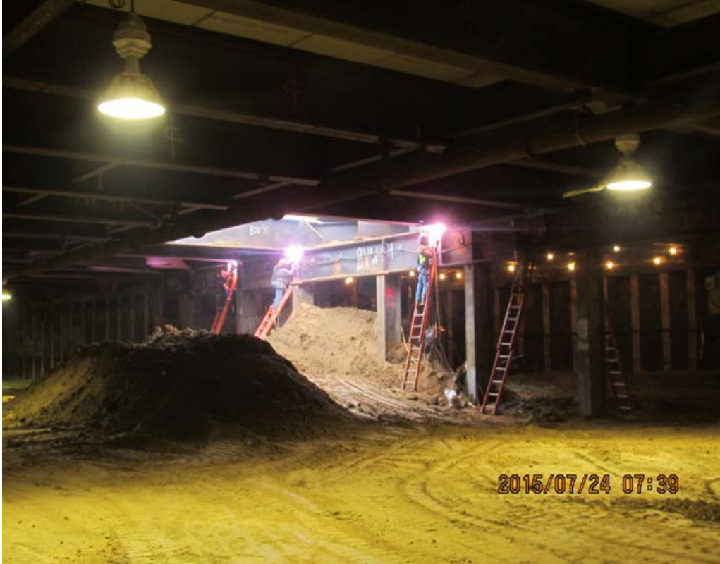
VERNON STATION - Welding of stiffener plates.
