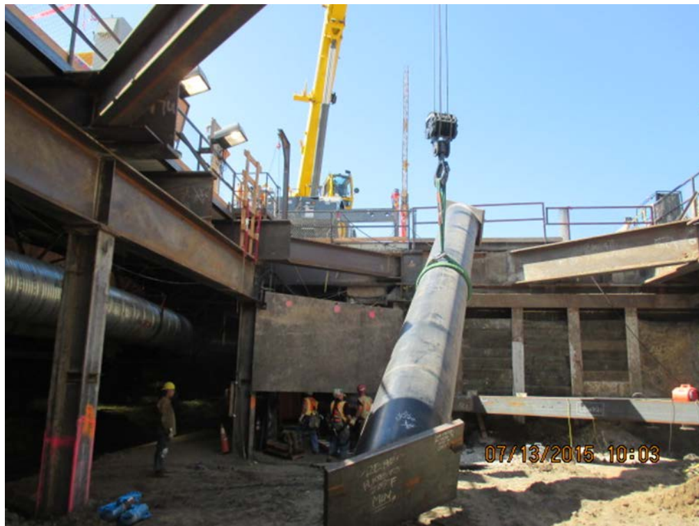
MLK STATION – Lowering of struts into the MLK station box.
