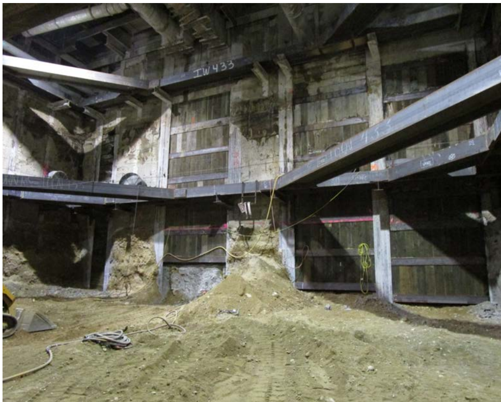
EXPOSITION STATION – Timber lagging operation at south headwall.
