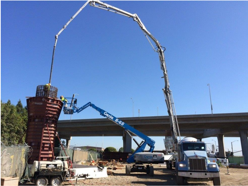
GREEN LINE - Underpass Bent 2A Column Concrete Placement.
