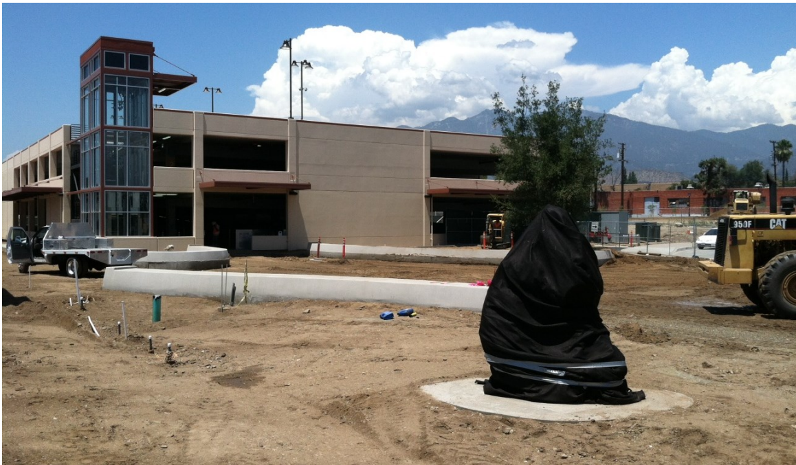
Monrovia Parking Structure Site Overview
