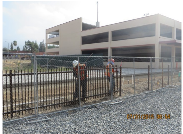
Segment 3: Monrovia Station - Picket Fence Installation
