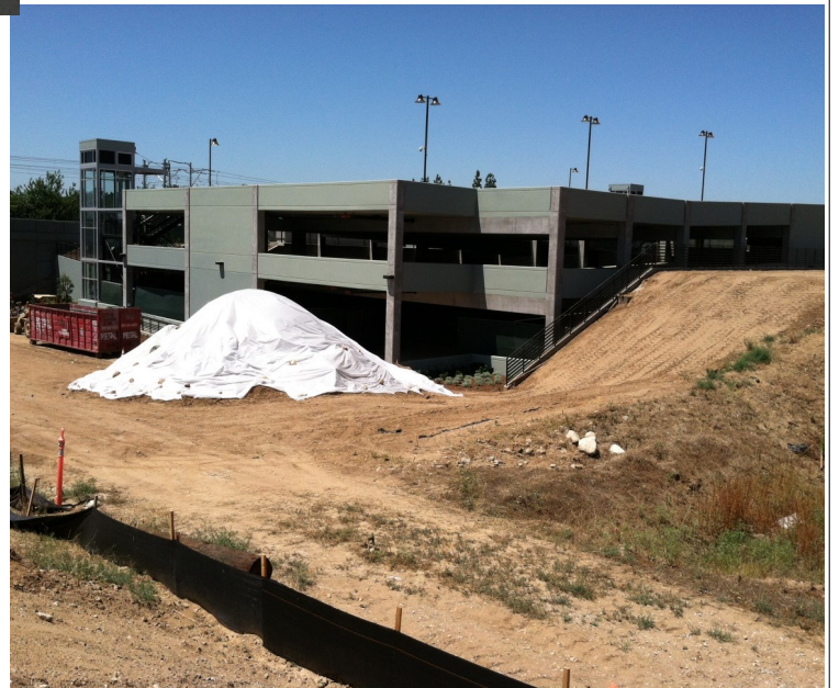
Azusa-Citrus Parking Structure Site Overview
