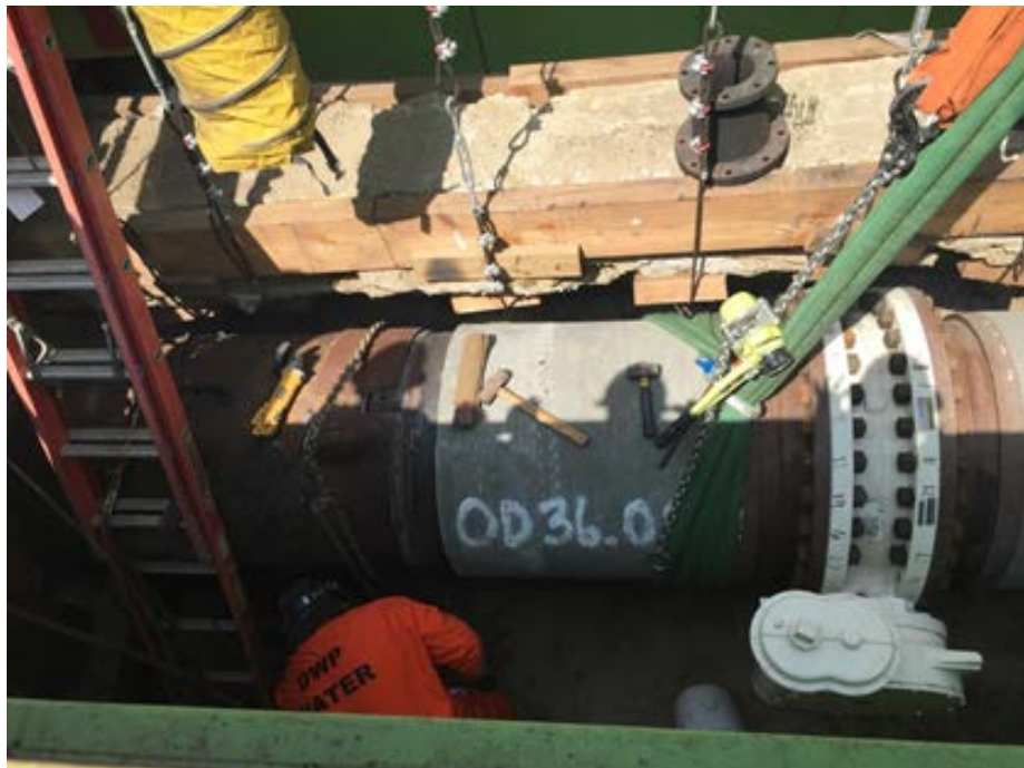
C0980 – 36" water valve installation at 1 st and Alameda
