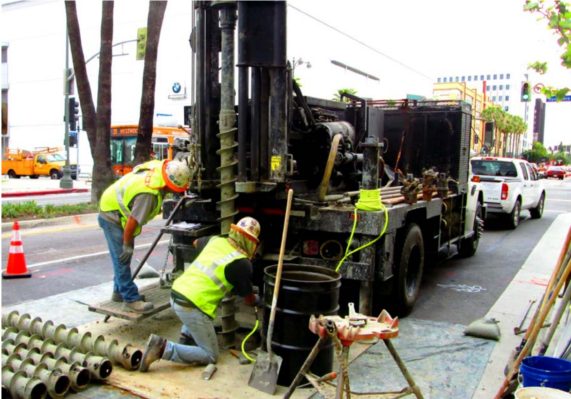
Geotechnical Site Investigation Work by the C1045 Contractor
