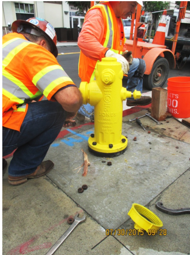
Buy America Fire Hydrants for Wilshire/La Brea and Wilshire/Fairfax
