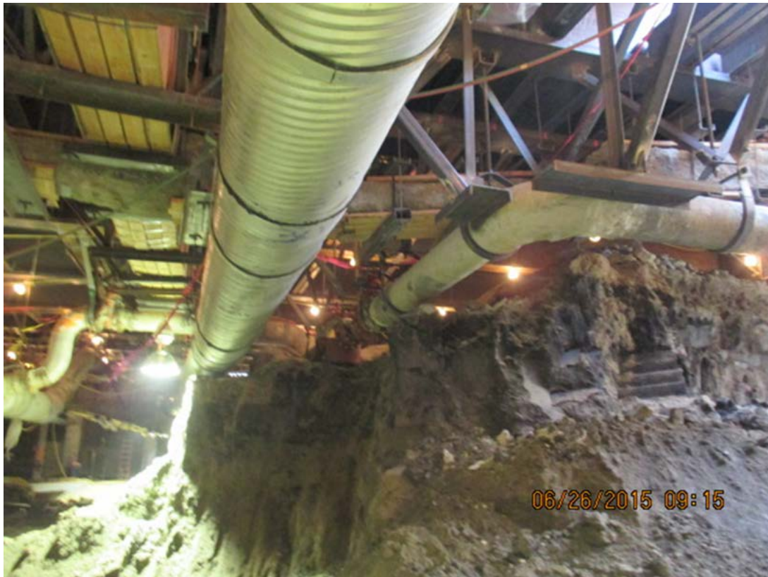
MLK STATION –Excavating under DWP fire line.
