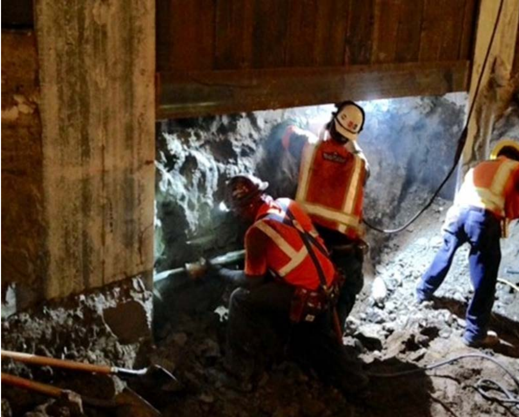
MLK STATION – Installation of timber lagging along the west wall.
