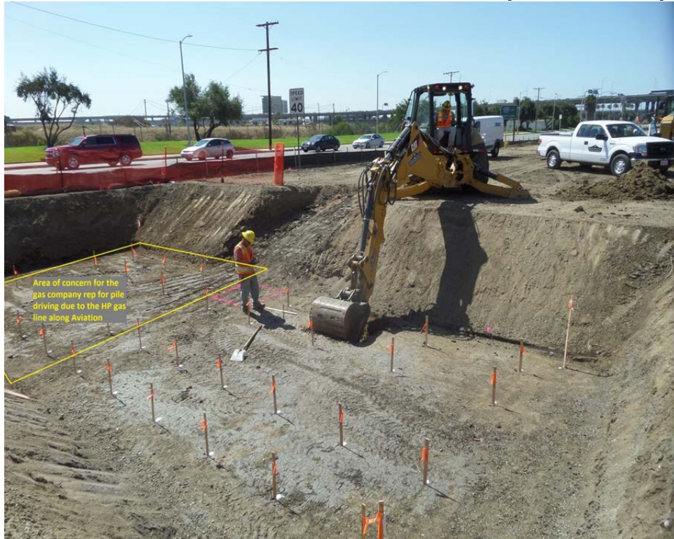
111 th street bridge - Excavating for PDA Piles Abutment 1 at 111 th Street.
