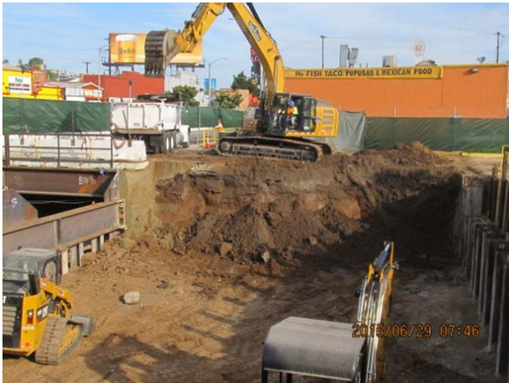
VERNON STATION - Looking north at the Excavation.
