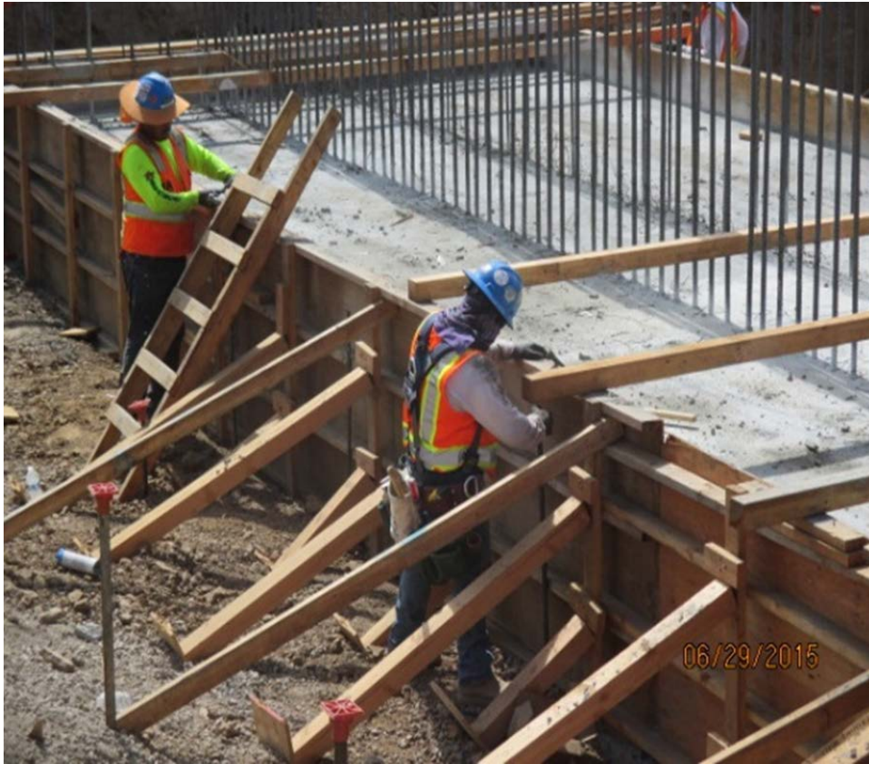
WSSC stripping forms from Imperial Abutment 10 Footing.
