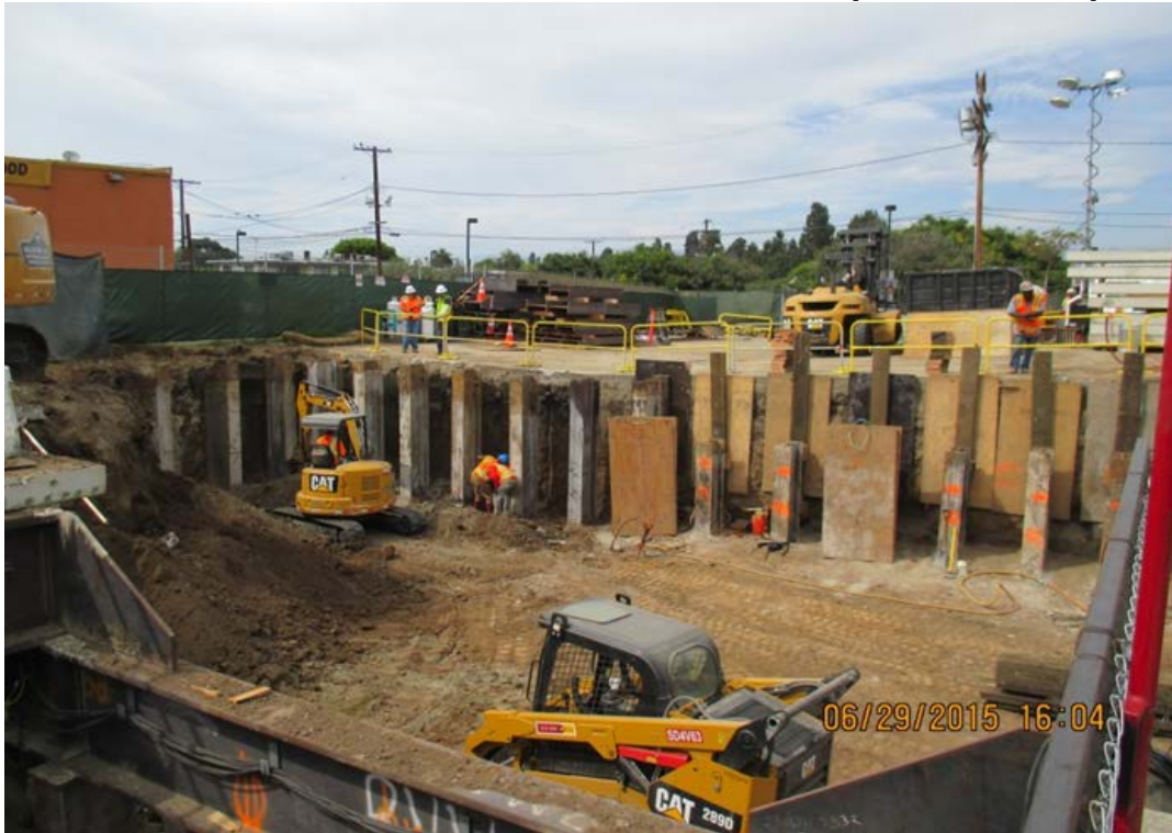
VERNON STATION – Excavation.
