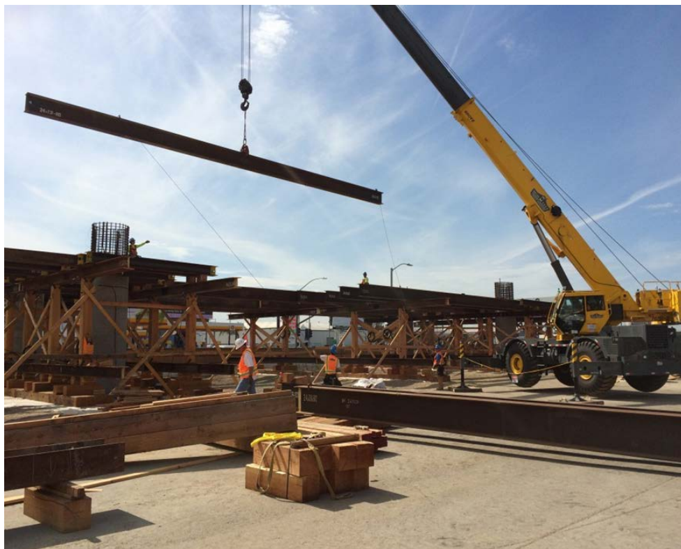
Aviation Century Underpass Stringer Beam Placement in Span 4.
