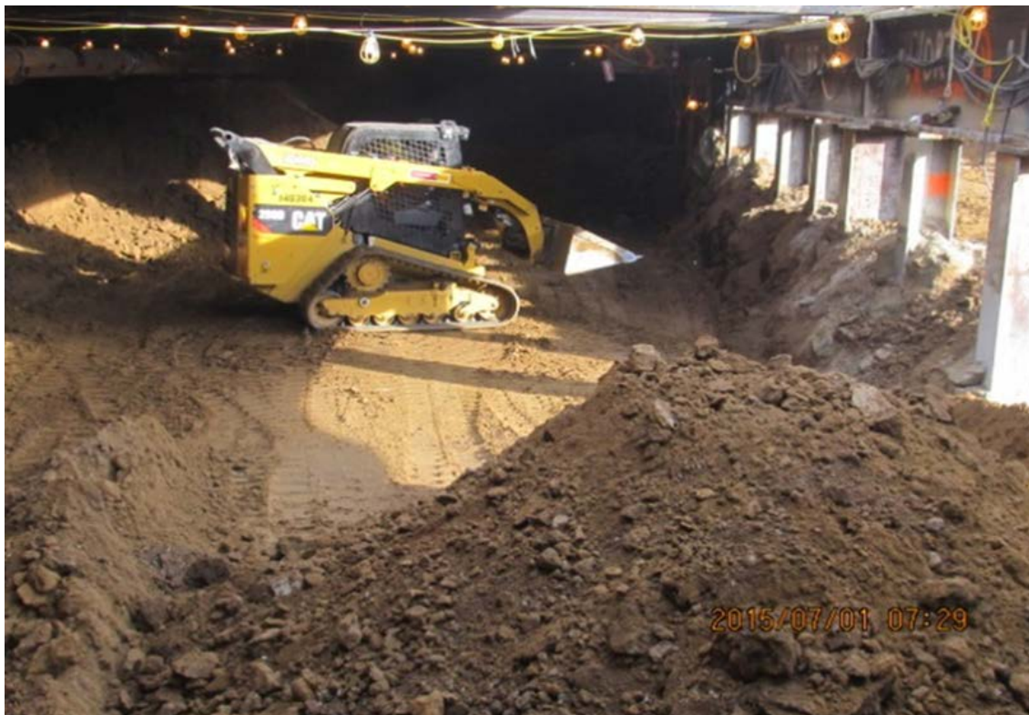
VERNON STATION - Excavation below Deck.
