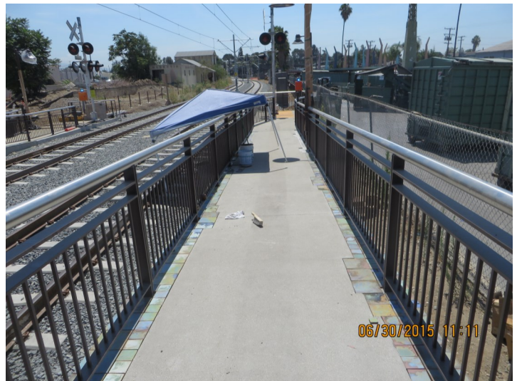
Segment 3: Monrovia Station - Quarry Tile
