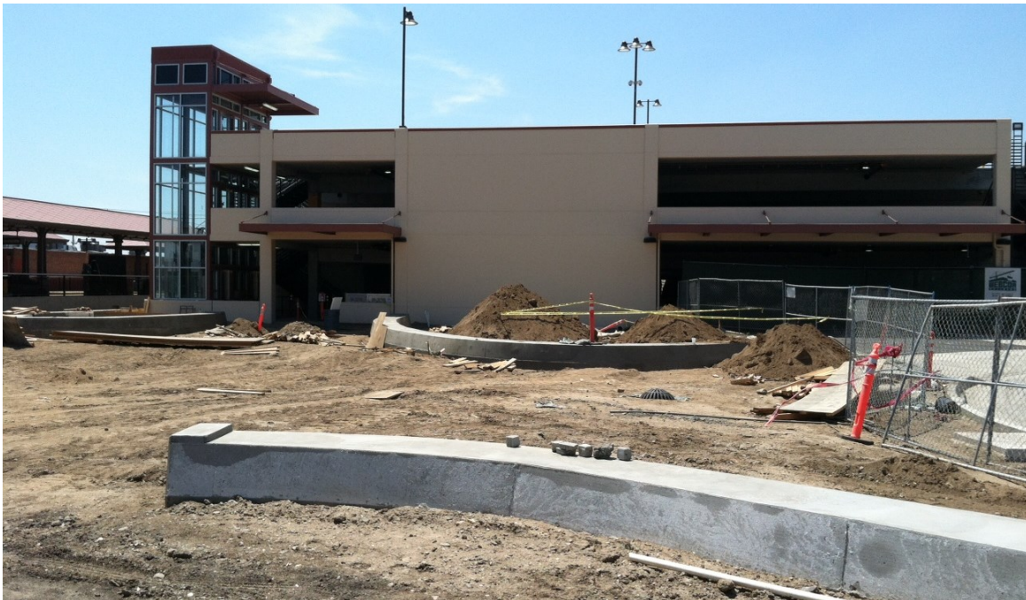
Monrovia Parking Structure Site Overview
