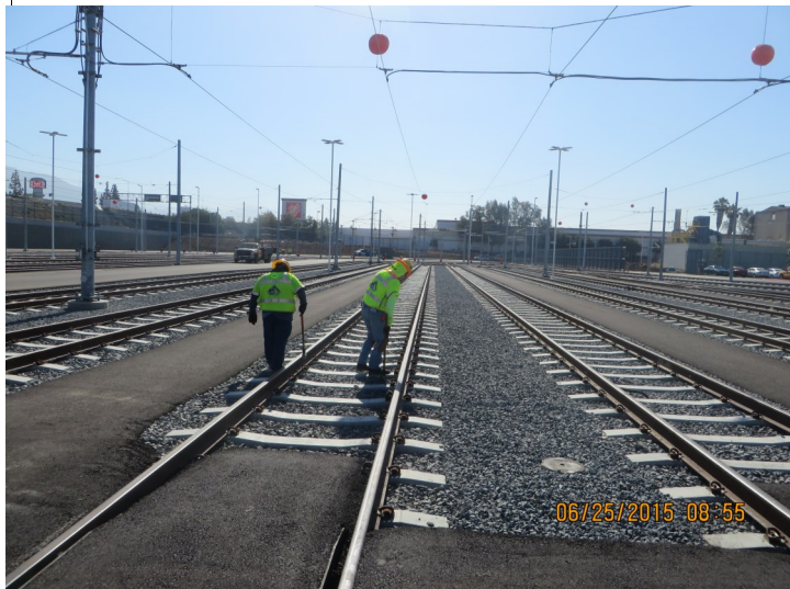
Operations Campus: Track Punch List Work
