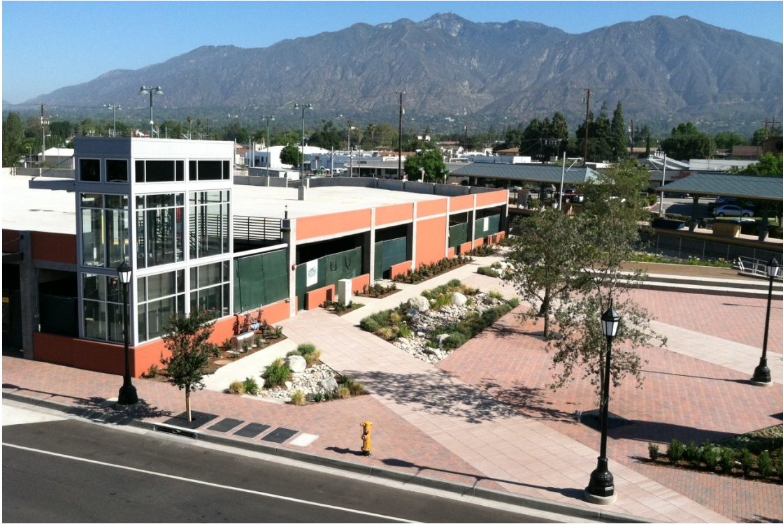
Arcadia Parking Structure Site Overview
