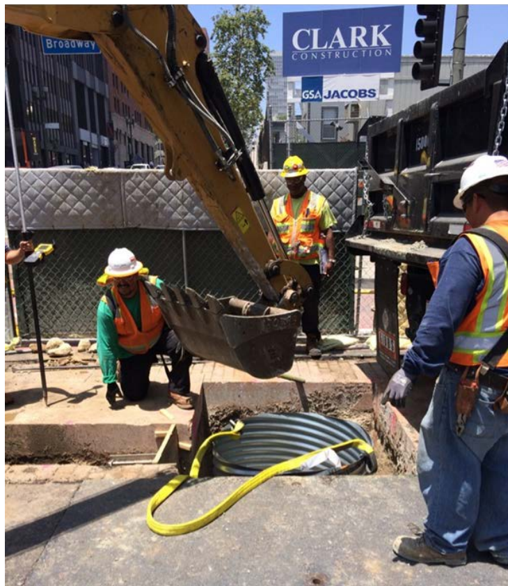
C0980 – Placing casing in Pile trench line at Broadway
