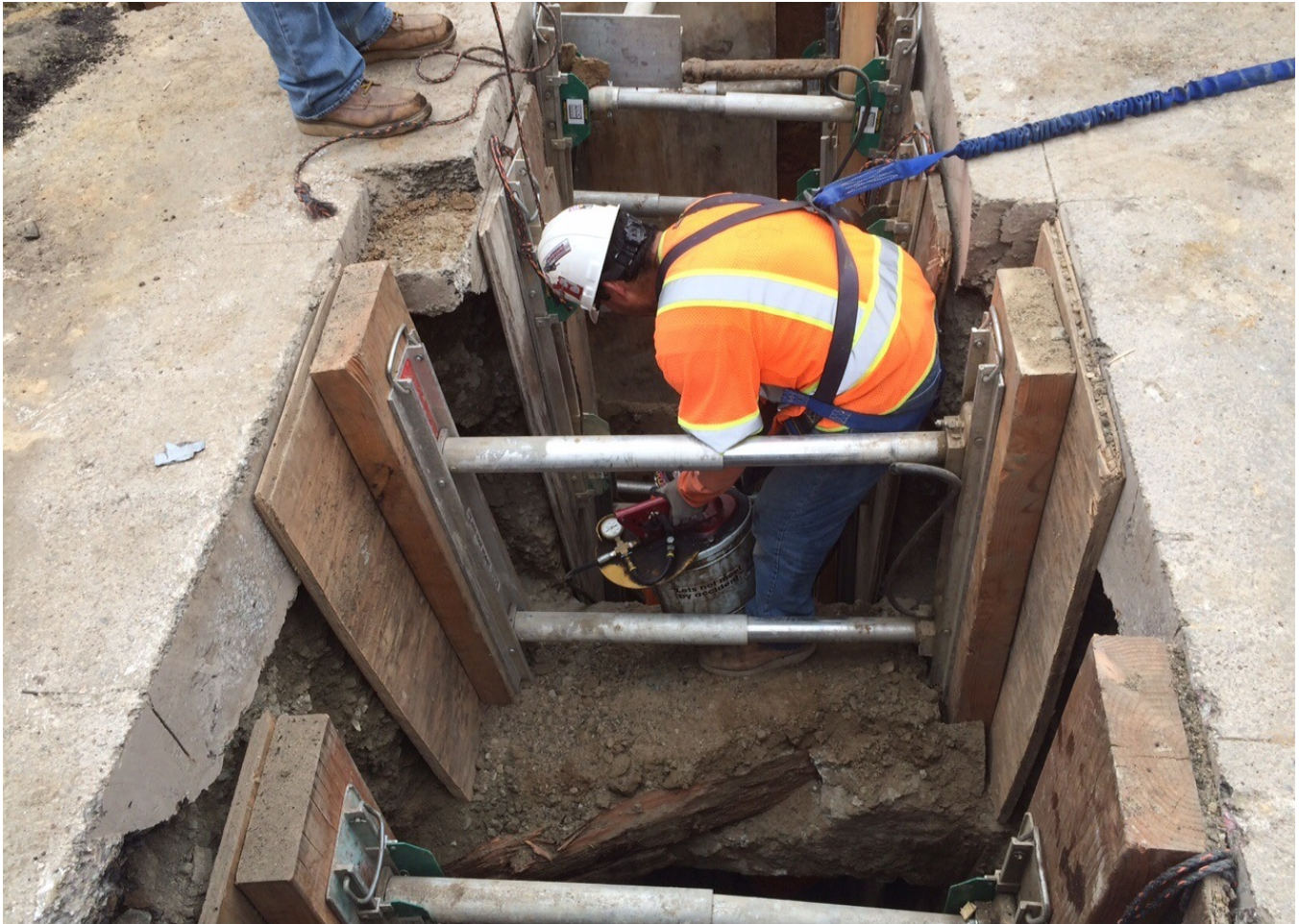
C1055 Wilshire/Fairfax AUR Placement of Trench Shoring
