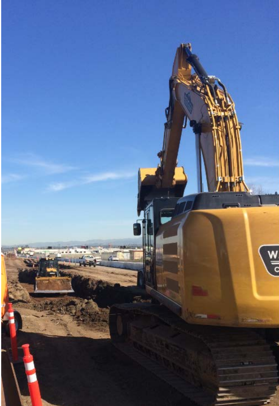
UG#1 Preliminary Excavation in Zone 3.
