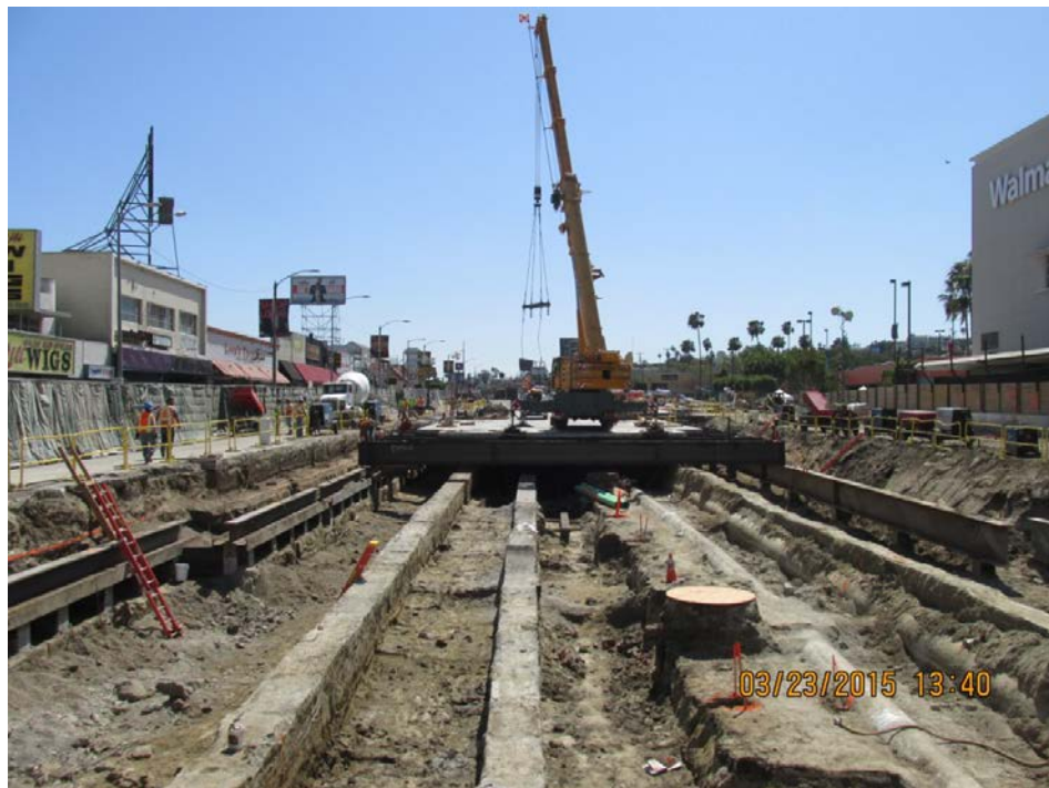
MLK Decking Operations.
