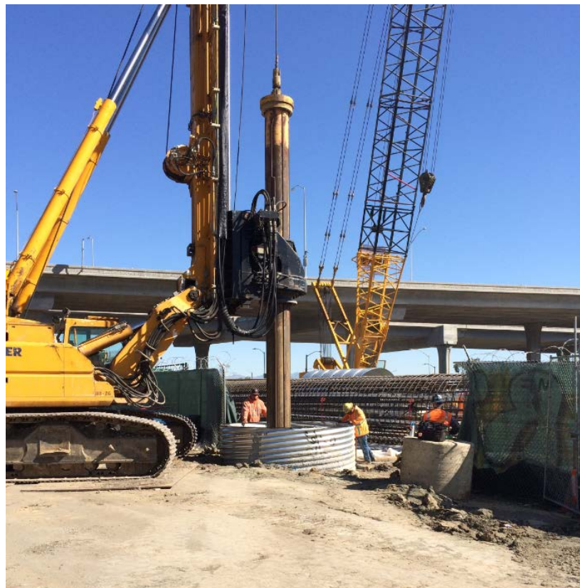
Green Line Underpass Drilling for Isolation Casing at Bent 2A.
