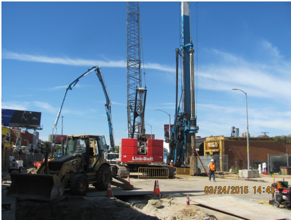
Vernon Piling Operation.
