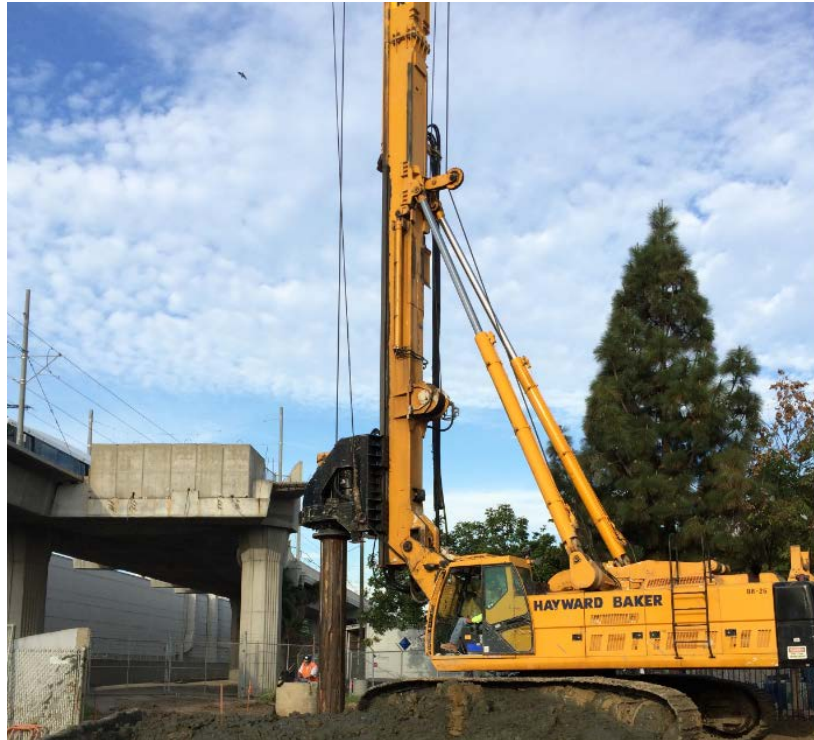
Green Line Bridge Bent 1A CIDH Safety Can Drilling.
