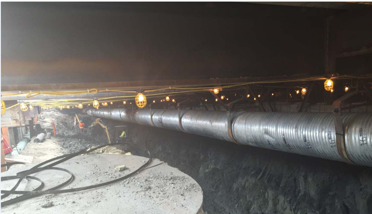
Temporary Support of Storm Drain at Exposition Station.
