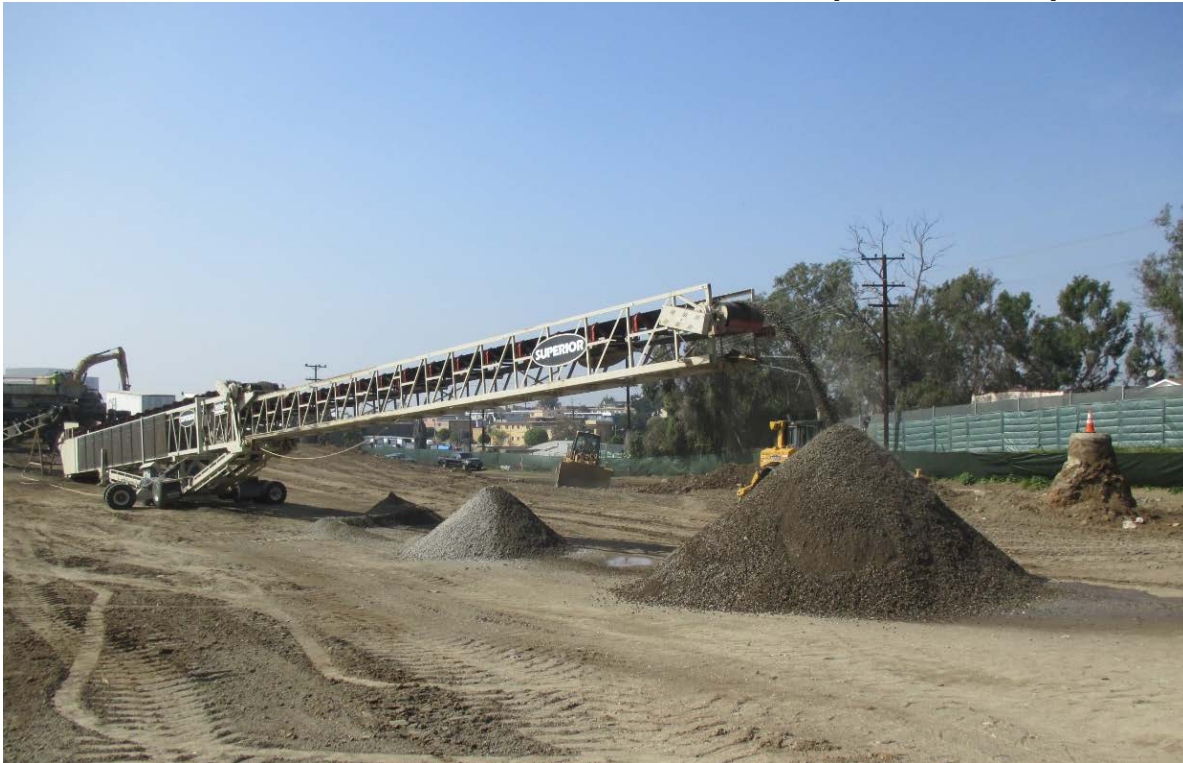
Stock Pile of the Recycled Concrete from the old Century Bridge demolished in July, 2014.
