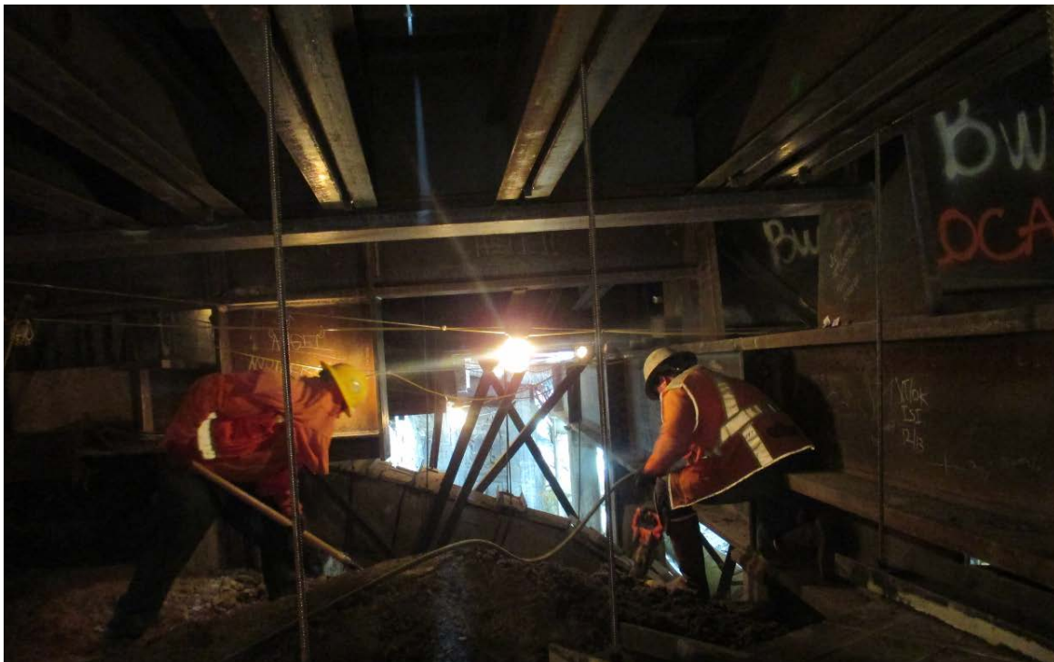
Soil Removal at Hobas Pipe at Exposition Station.
