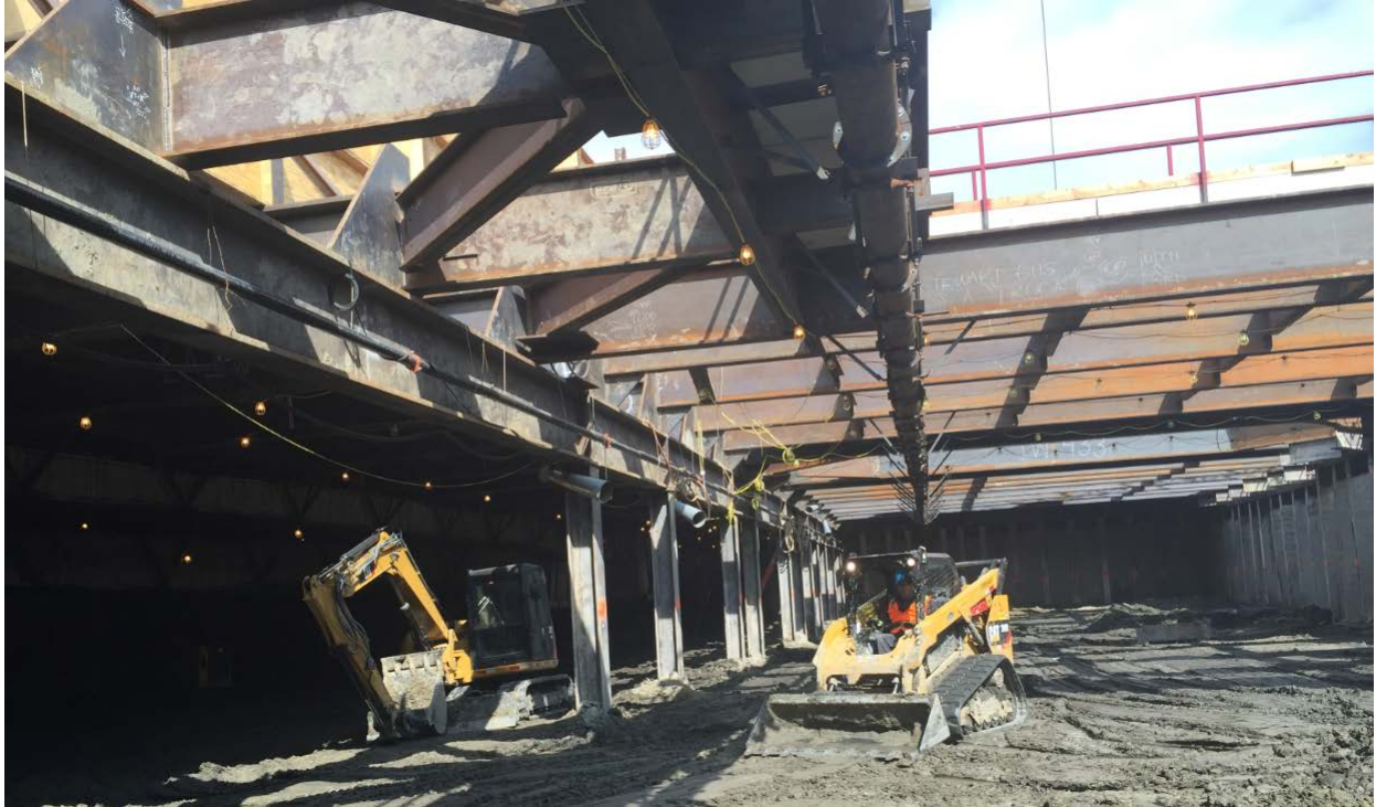
Soil Grading at -21 Feet Level Prior to Installation of Bracing.
