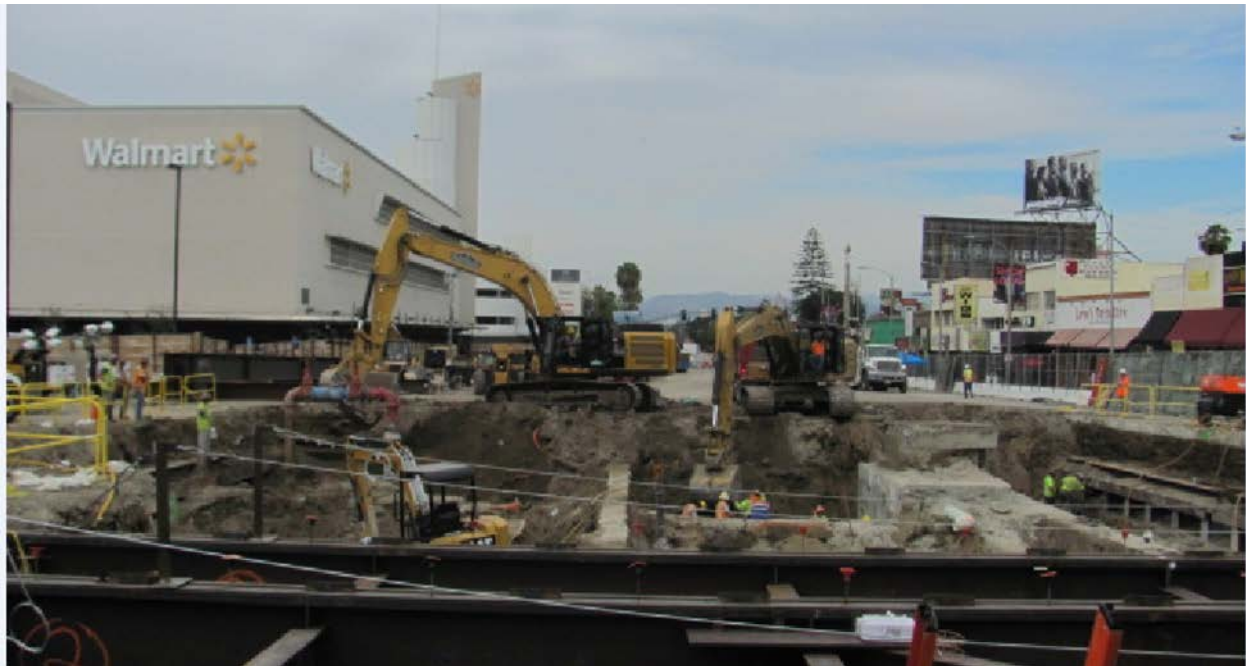
Excavation for Decking at MLK.
