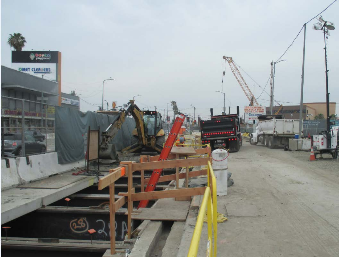
Soil Removal at Beam 32-33 at Exposition Station.
