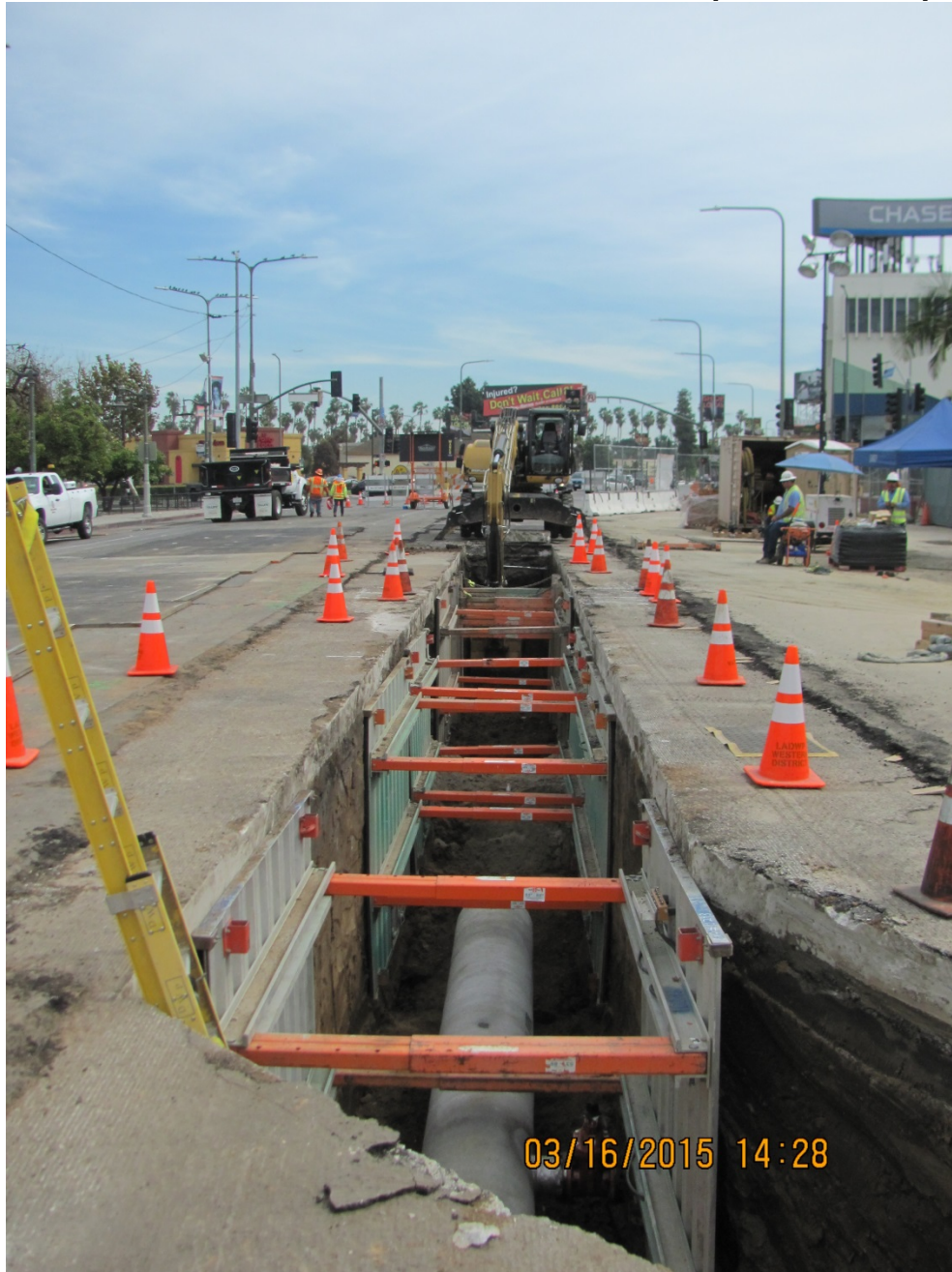
DWP Relocation of 24" Waterline at Vernon.
