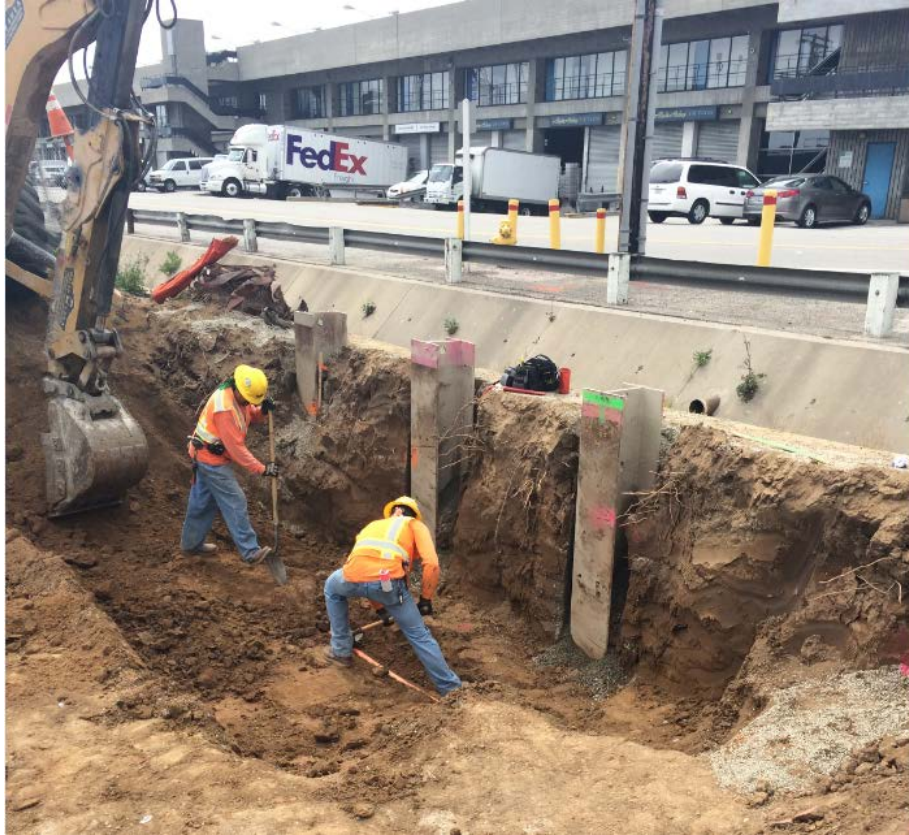
Century Aviation Aerial Structure Abutment 1 Excavation for Qwest Line Relocation.
