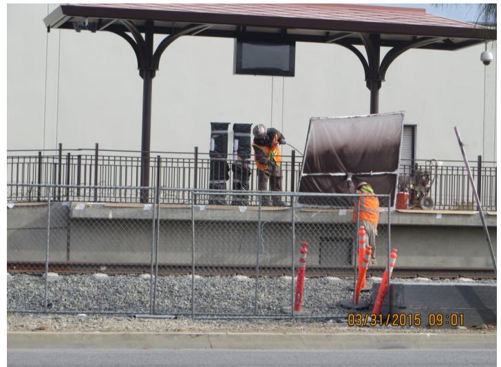
Segment 3: Duarte Station - Guardrail Painting
