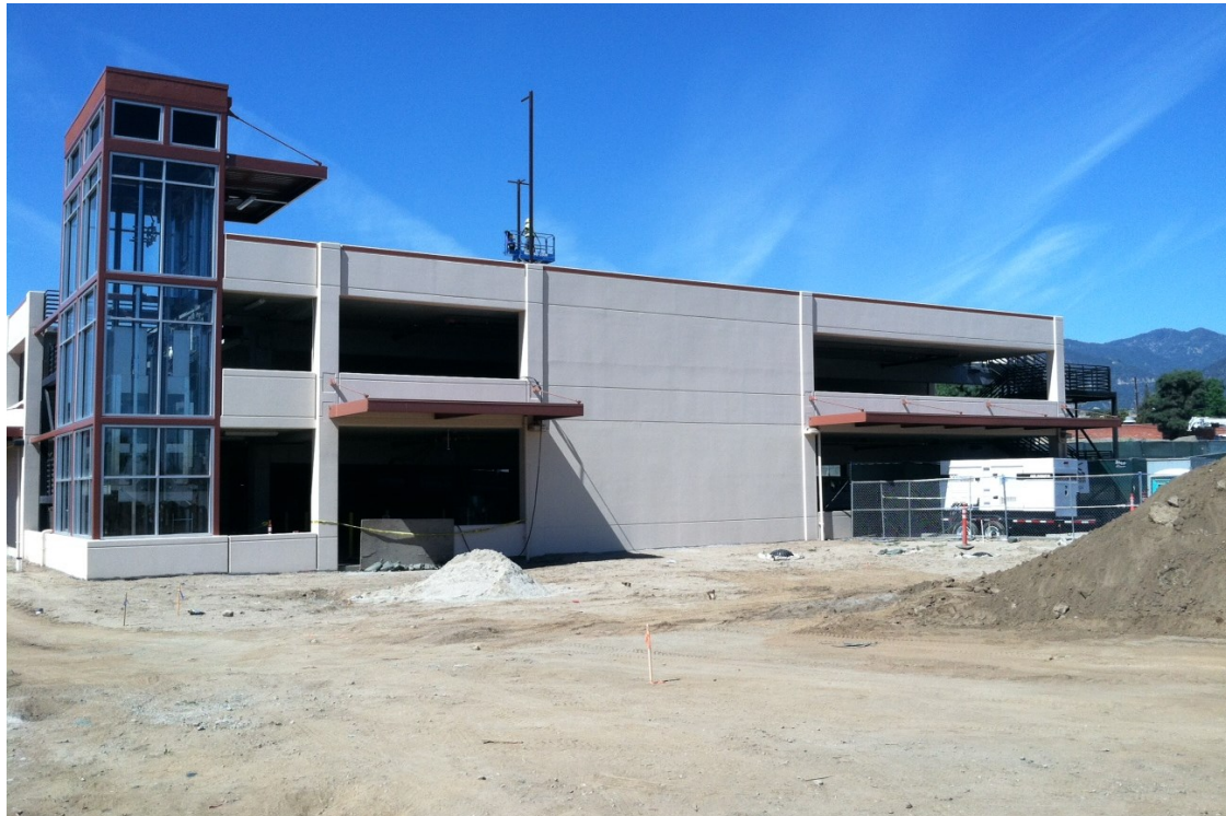
Monrovia Parking Structure Site Overview
