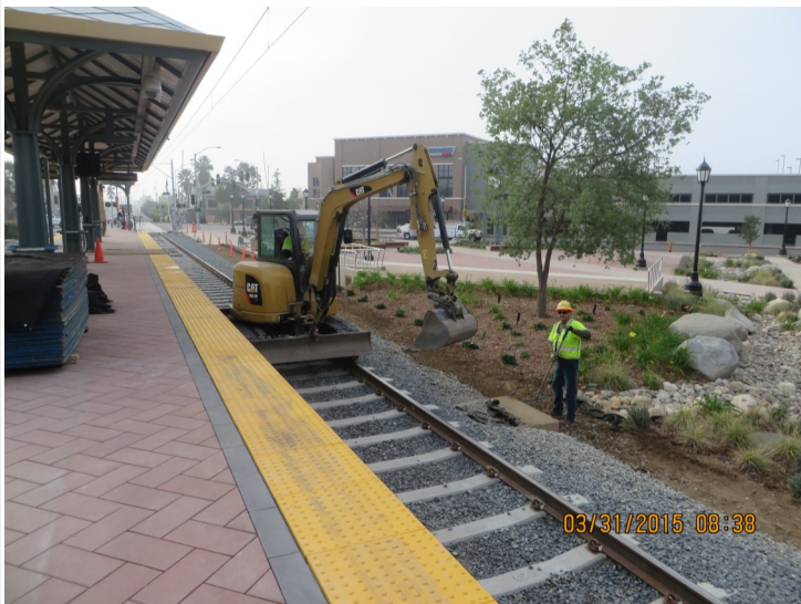
Segment 2: Arcadia Station - Grading Work
