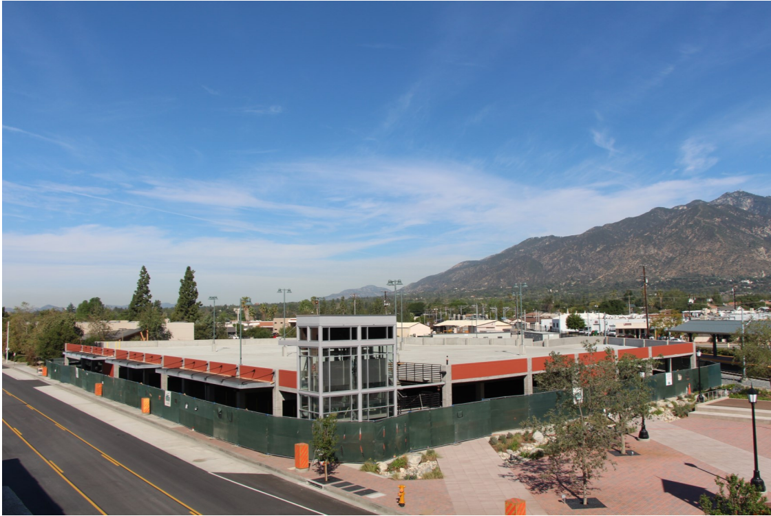
Arcadia Parking Structure Site Overview
