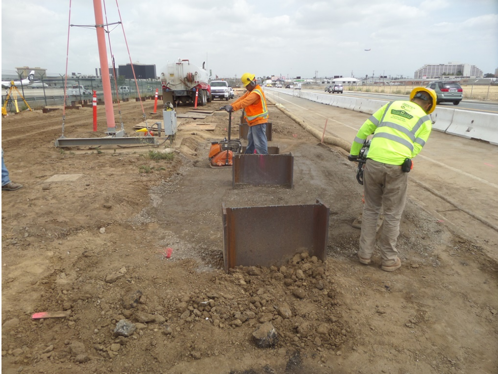
WSSC Placing and Compacting CMB for Navaid Light Footer.
