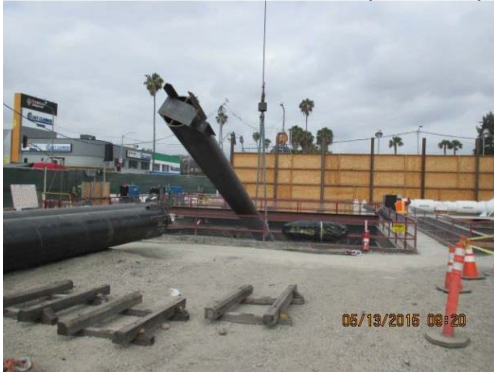
Hoisting Strut Down the Expo Shaft.
