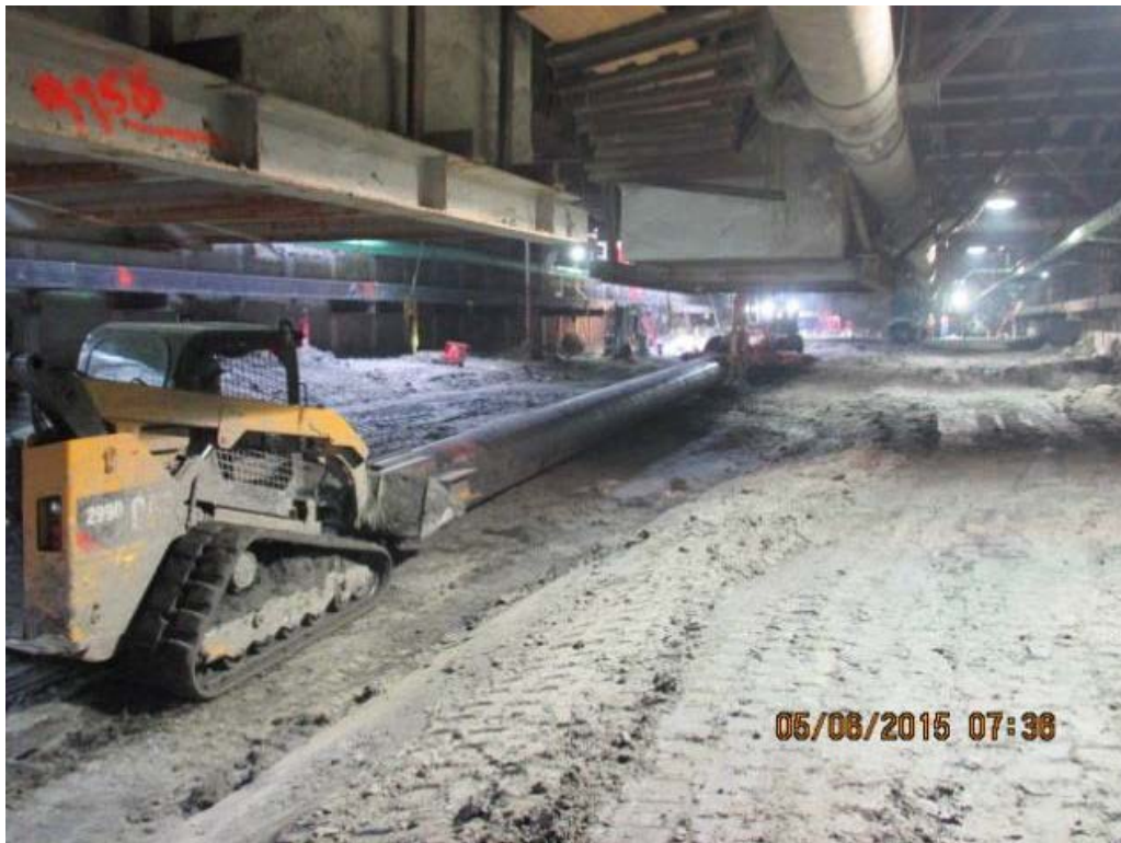
Dragging Struts to South End at the Expo Station.
