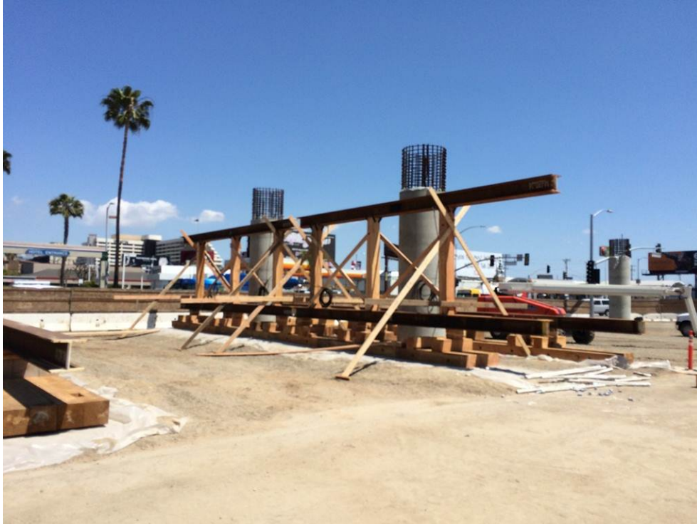
Aviation Century Underpass Falsework Bent 5-1.
