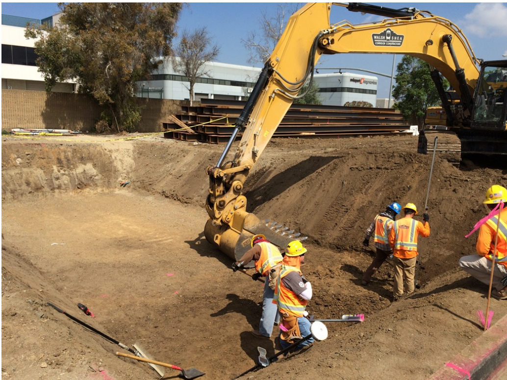
111 th Street Underpass Abutment 2 Footing Excavation.
