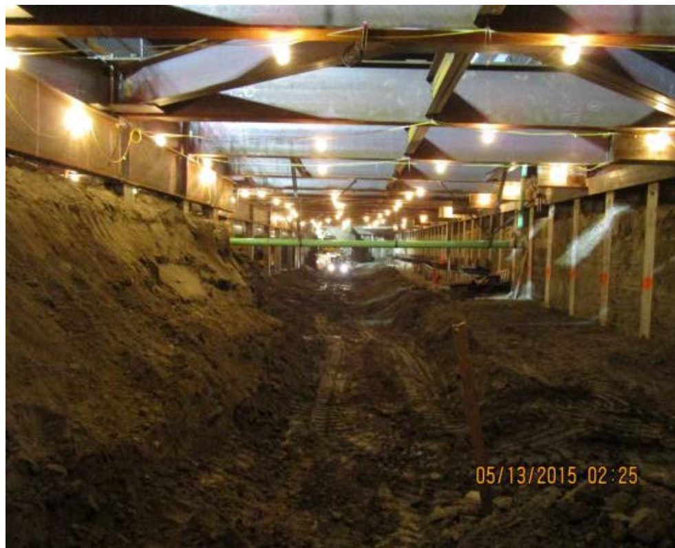
Excavation in the Northwest Station Box at MLK.
