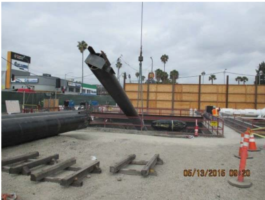
Hoisting Strut Down the Expo Shaft.
