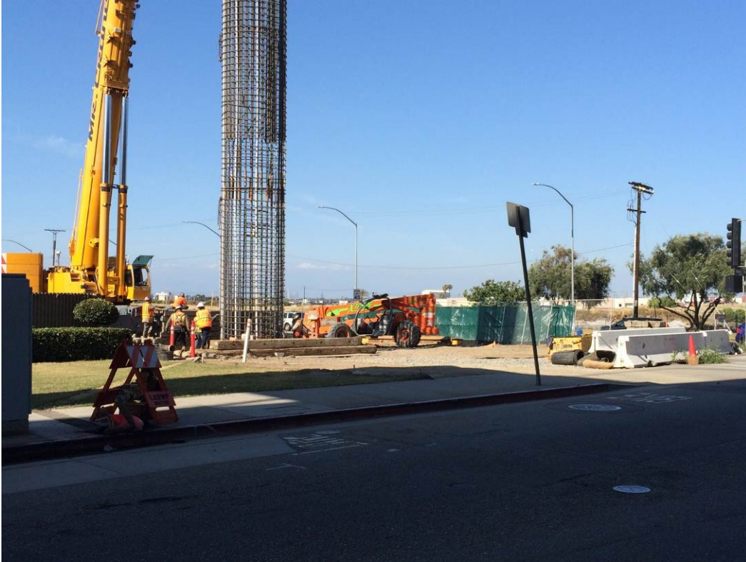
Green Line Underpass Bent 5 Column Rebar Cage Placement.
