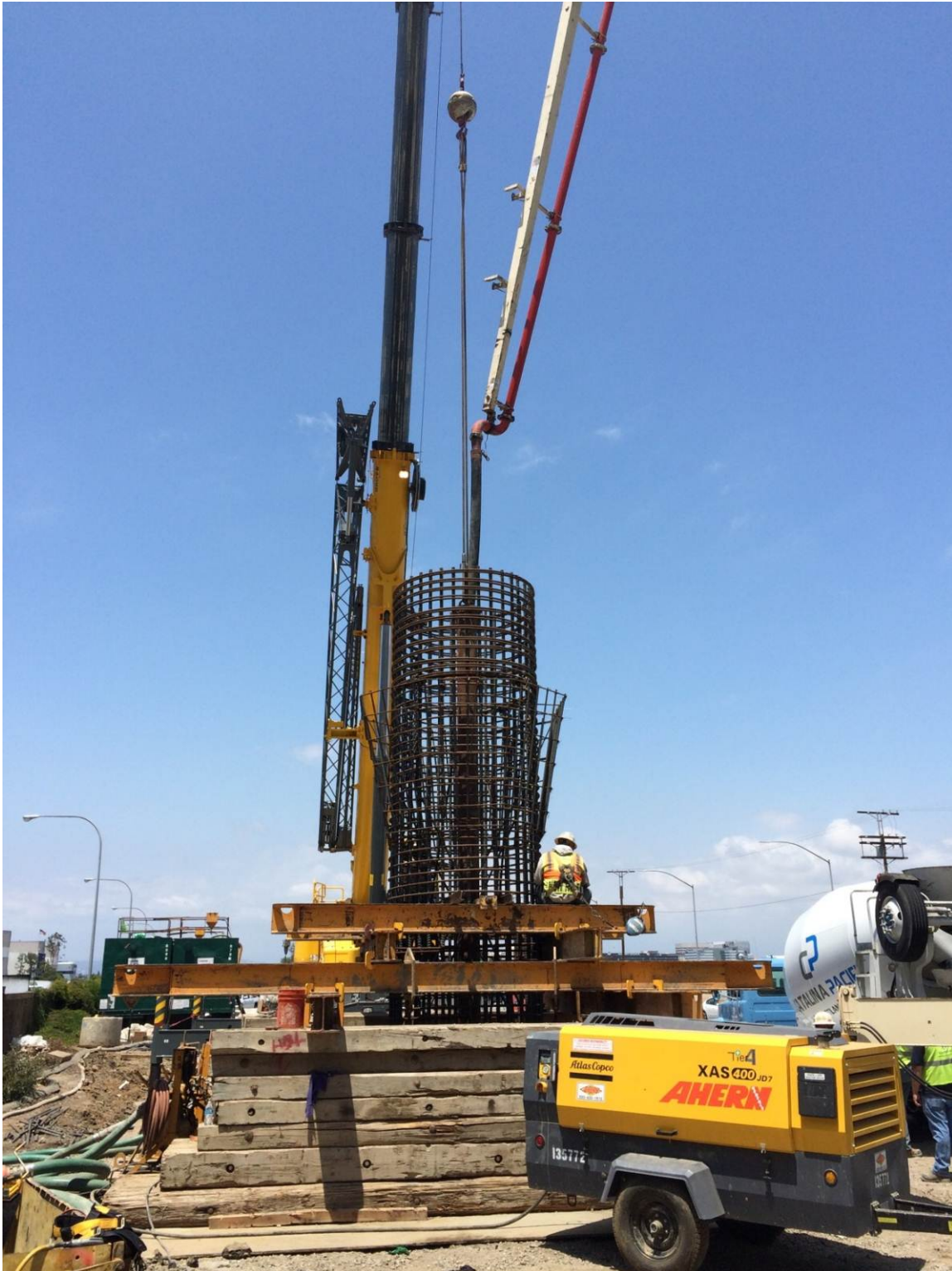
Concrete Placement for CIDH #5 (Bent 5).
