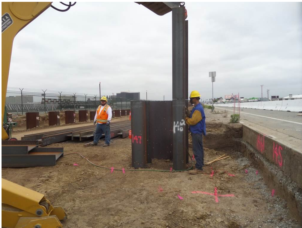
Topping SOE Piles at Emergency Stair Case 2.
