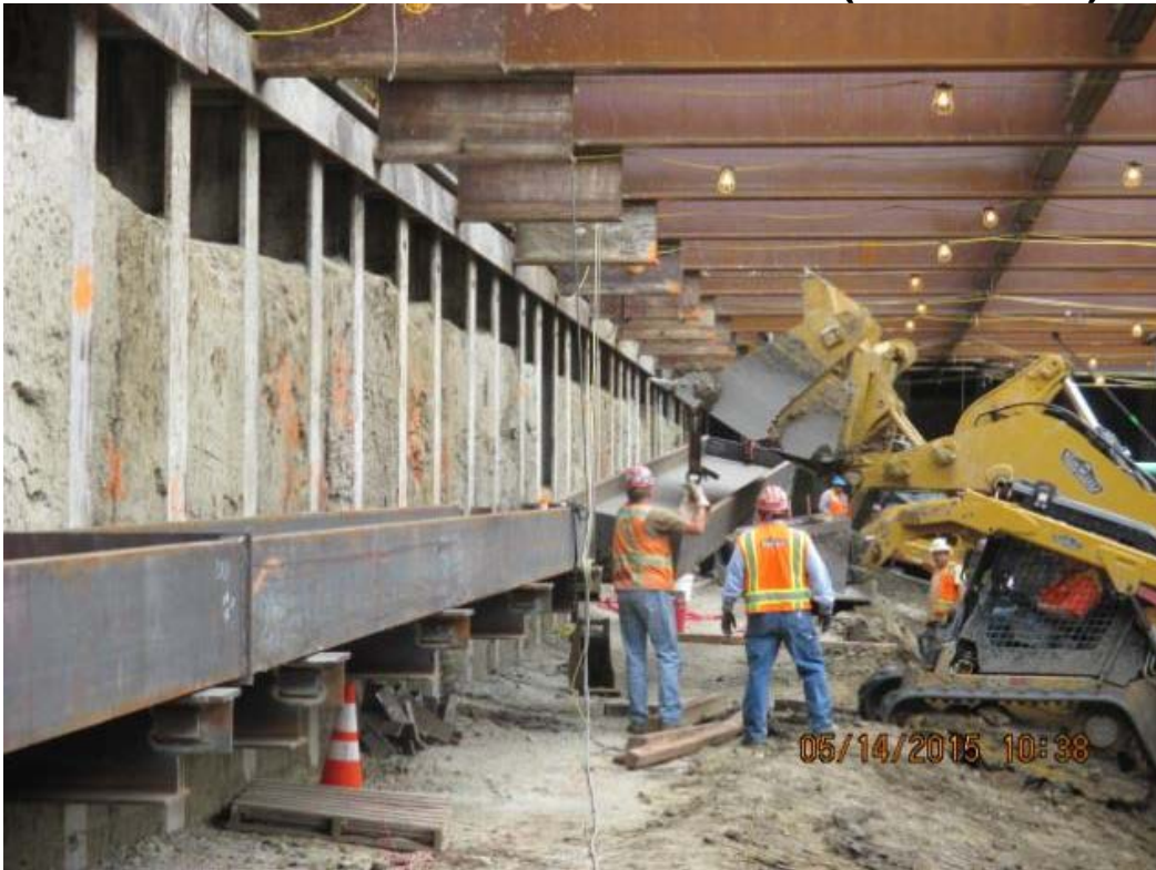
Installing West Walers at the MLK Station.
