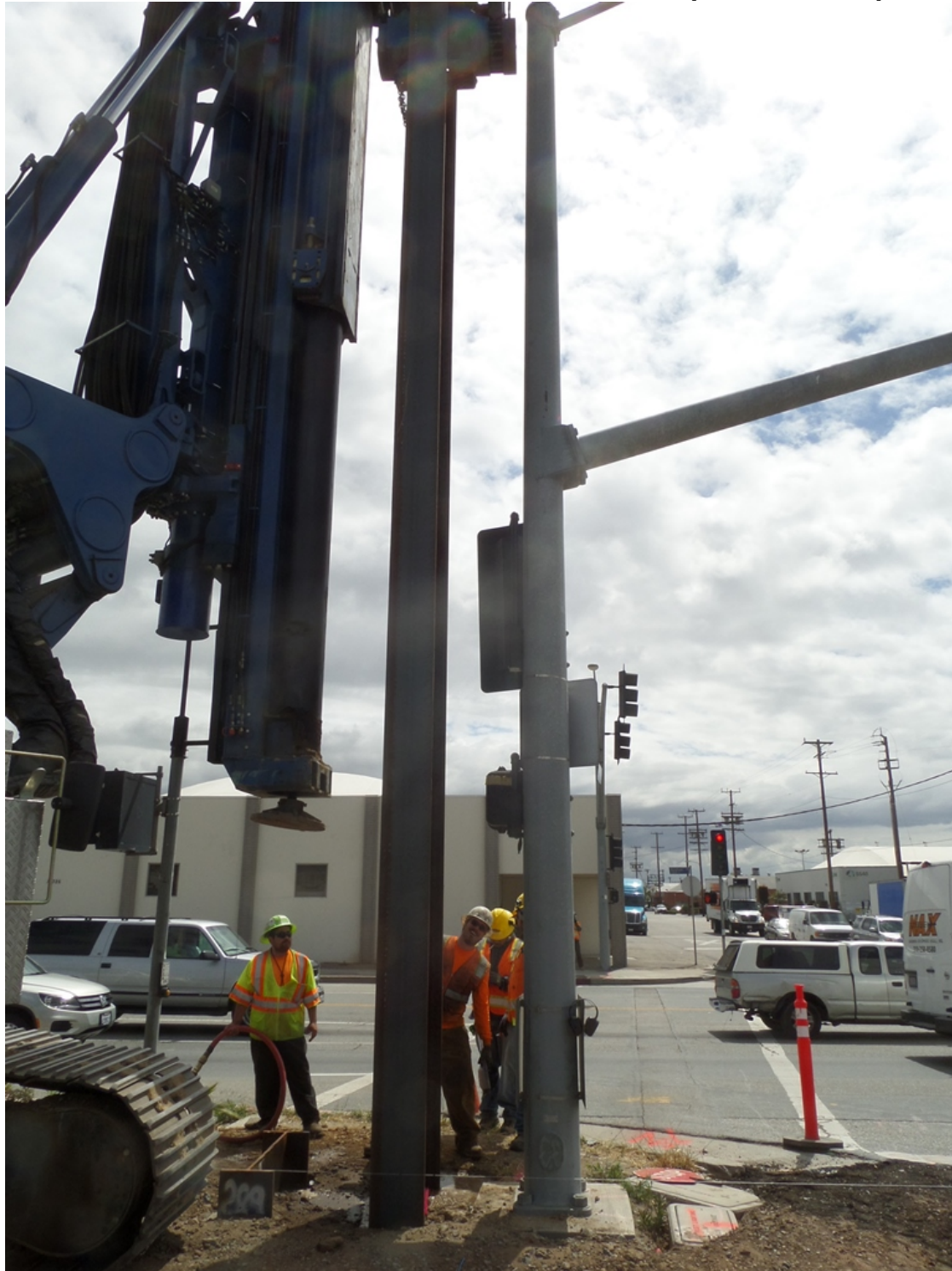
Installing SOE Pile 288.2 North of 104 th Street.
