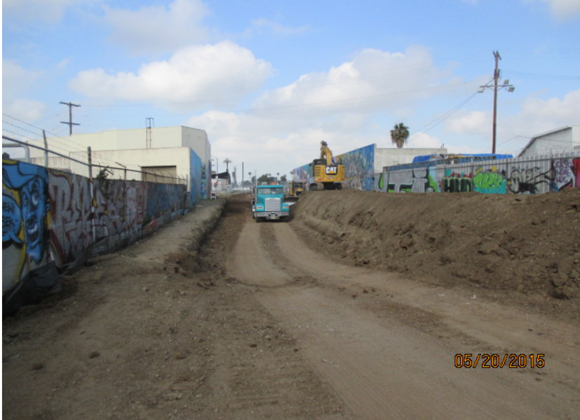
Pile Driving at La Brea Bridge Abutment 2 (East).
