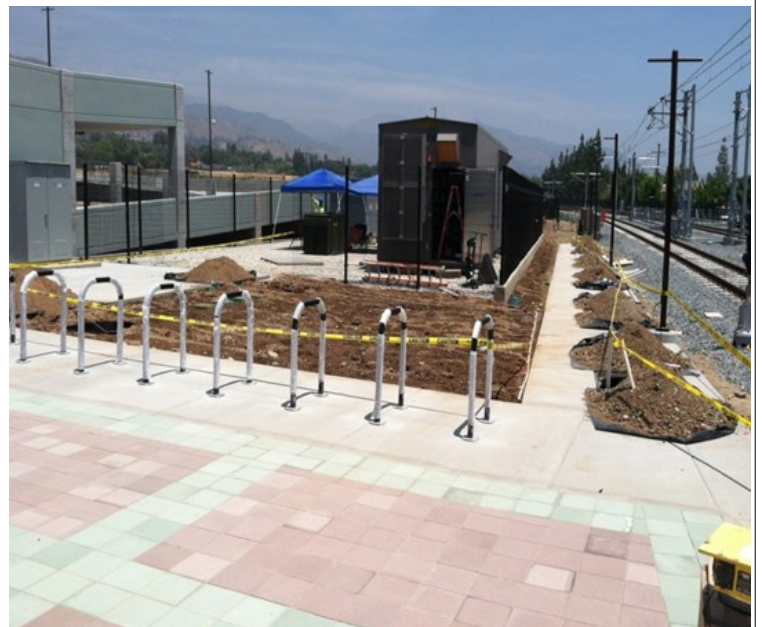
Azusa-Citrus Parking Structure Site Overview
