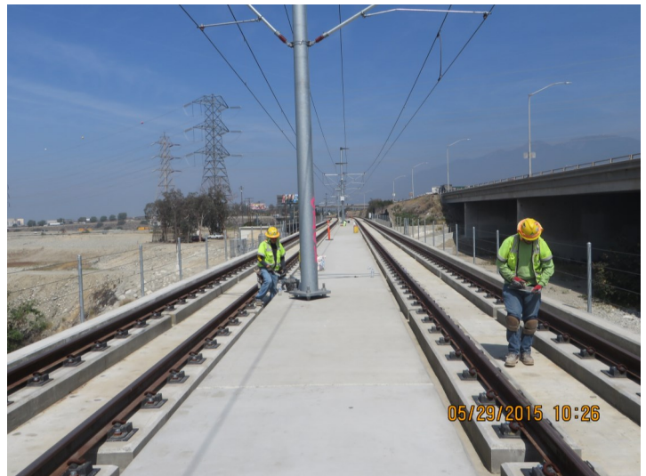
Segment 3: San Gabriel River Bridge - Concrete Punch List Work
