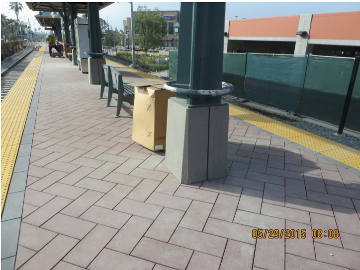
Segment 2: Arcadia Station - Column Bases
