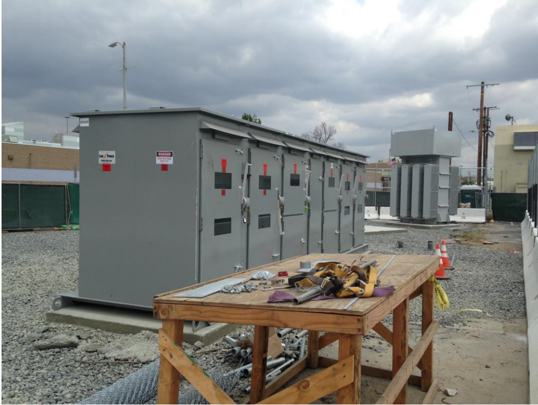
C0980 Contract – Substation at Mangrove Yard
