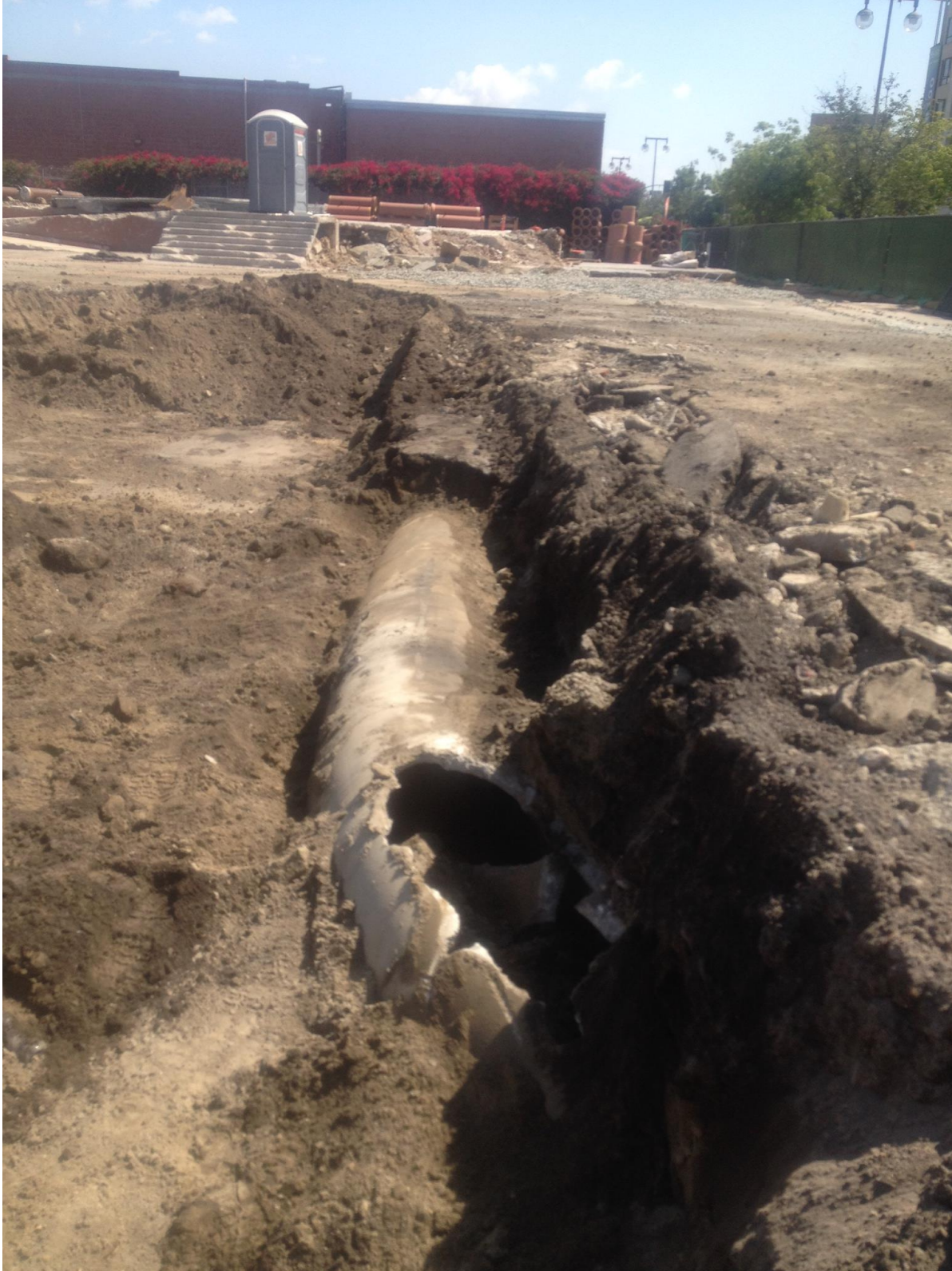
C0980 - Discovery of Zanja Segment at 1 st and central Station location
