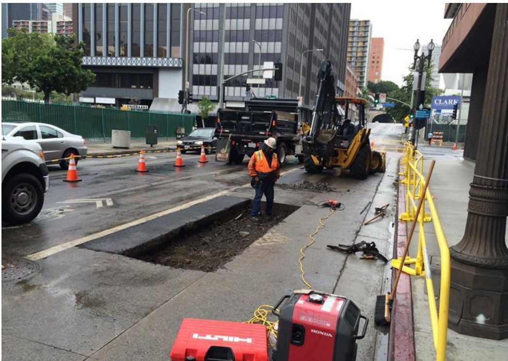
C0980 Contact – Pile Trenching on 2 nd Street
