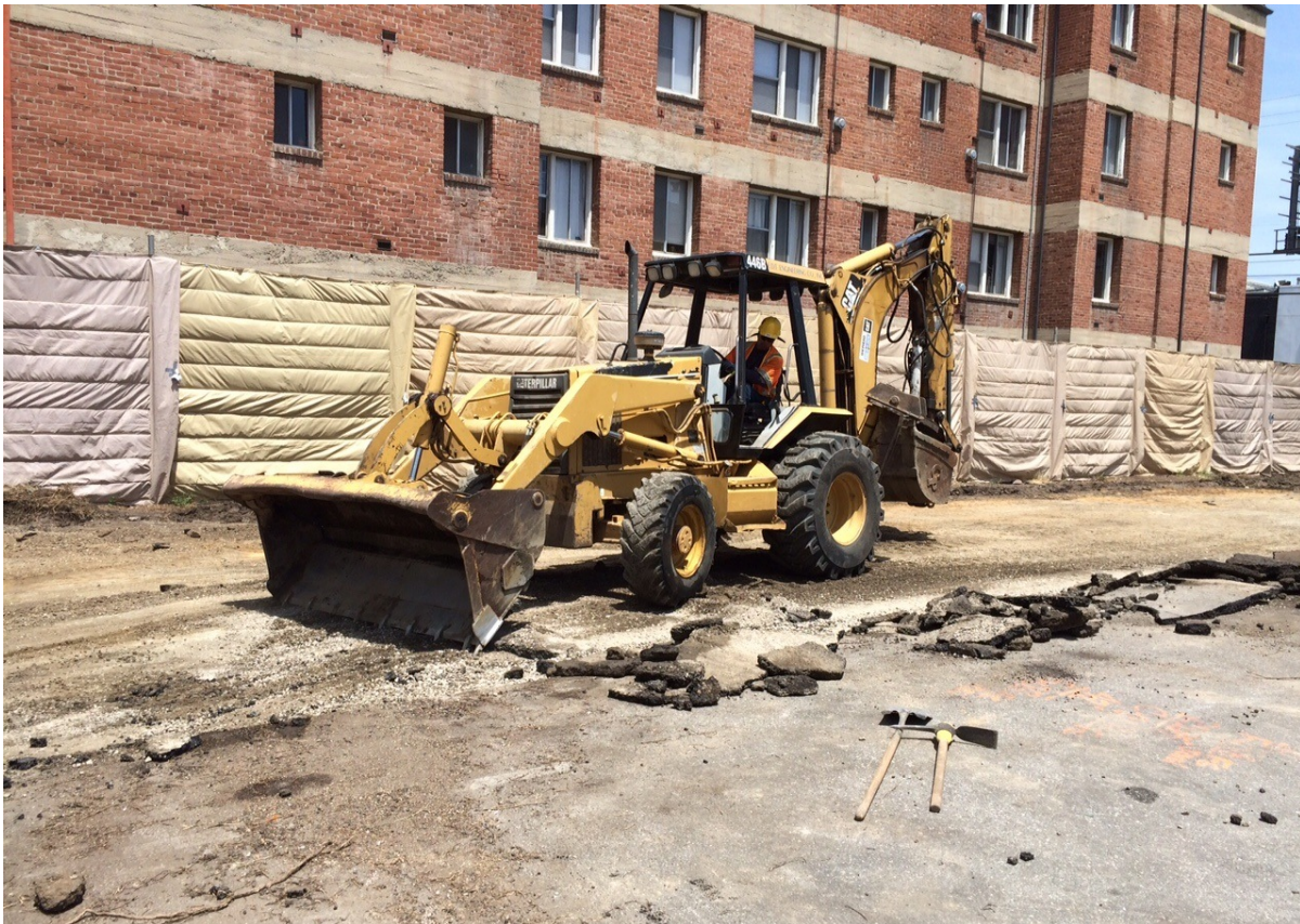
C1045 Design/Builder Site Preparation Work at Detroit Lot
